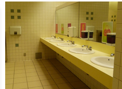
Figure 130- Existing Women's Washroom.
