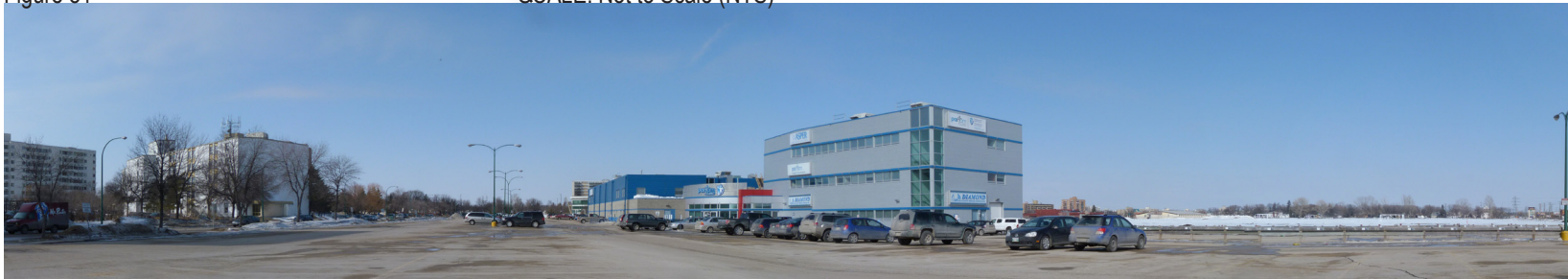
Figure 82 - View of Pan Am Clinic from Taylor Ave..
