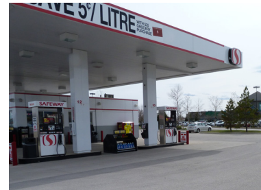
Figure 141 - Gas Station on Site.
