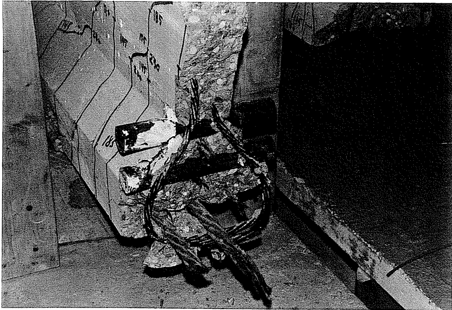
Figure 4.14 (a) Failure mode of beam TR-1-7.5/7
