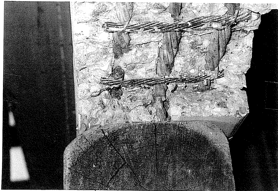
Figure 4.14 (c) Failure mode of beam TR-3-5/7
