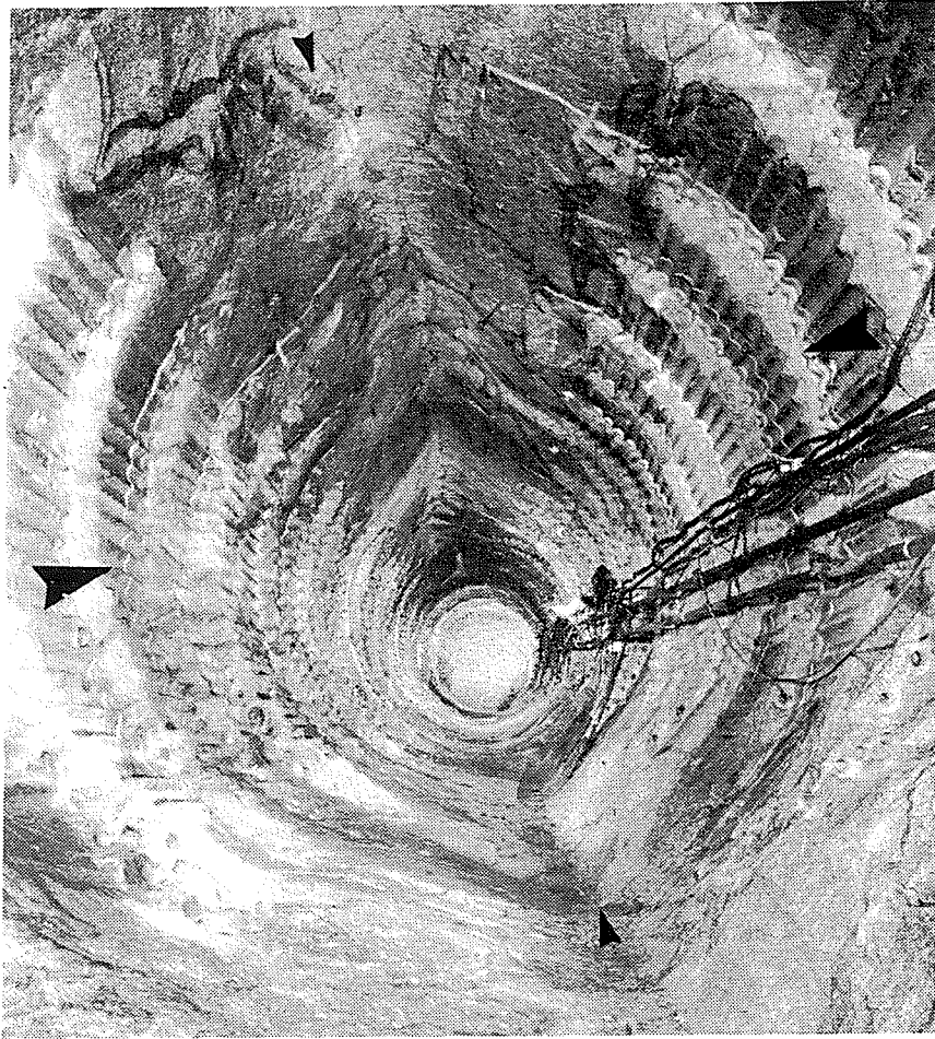
FIGURE 5.8: Breakout Notch Development In Situ in the Mine-by Tunnel. The breakout develops towards the minimum principal stress which is marked by the smaller arrows. Larger arrows indicate the maximum principal stress direction. Compare with Figure 5.7.
