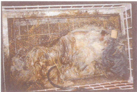
E. Advanced Decay
