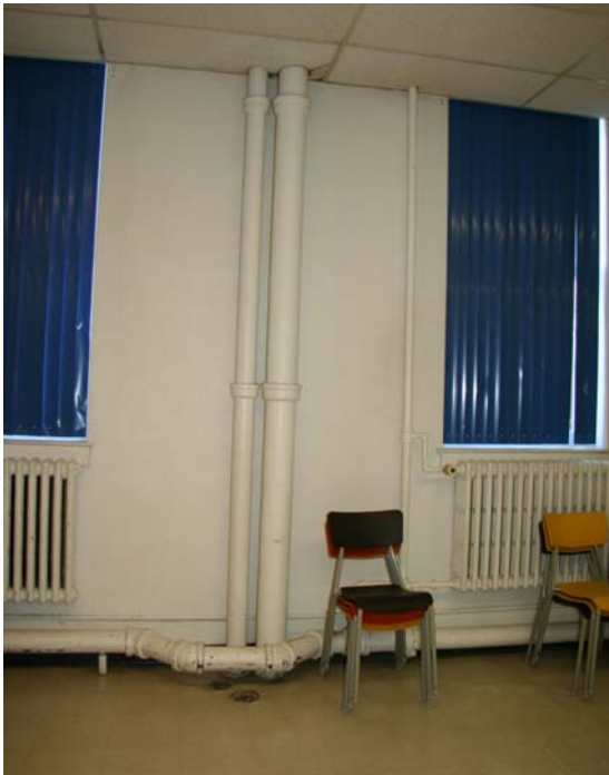
Figure 2.67. Sewer lines, located on the interior of the north façade at the center of the 1928 addition. Image by Natalie Foidart.
