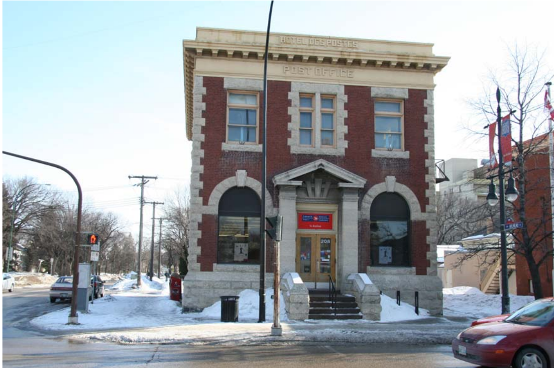
Figure 2.9. Original Saint-Boniface Post Office built in 1909, located on boulevard Provencher. Image by Natalie Foidart.
