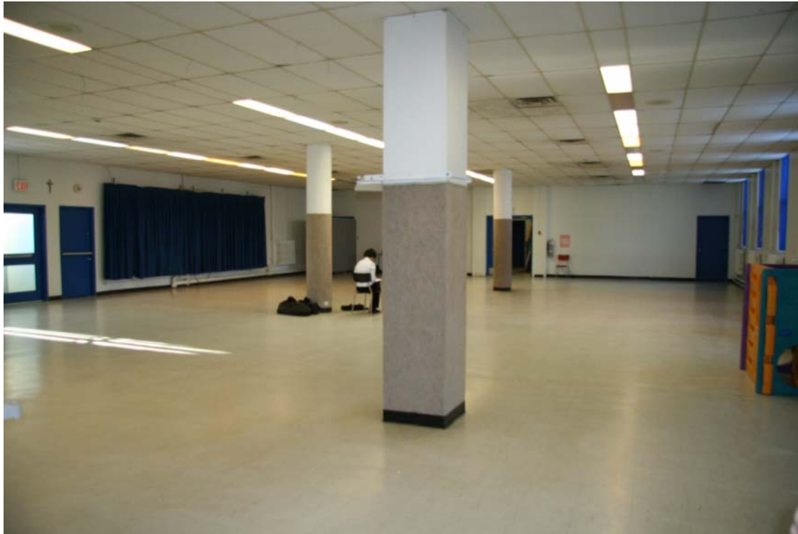
Figure 2.45. Existing open plan basement in the 1928 section of 210 rue Masson. Image by Natalie Foidart.
