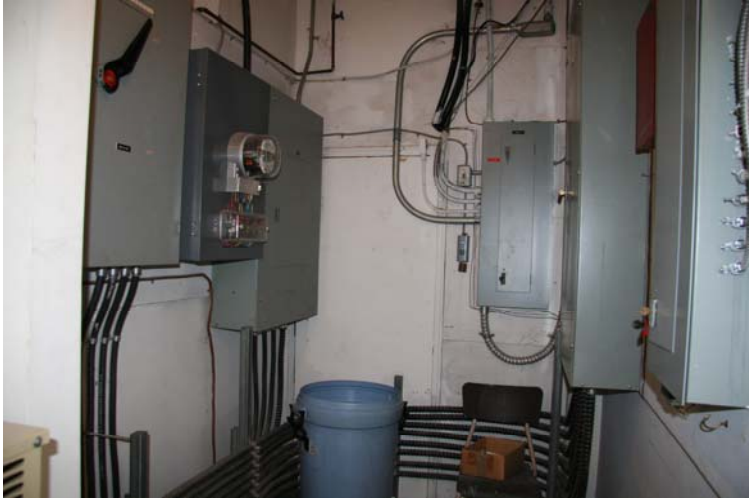
Figure 2.66. Electrical panels for the building, located in the northeastern corner of the 1928 addition. Image by Natalie Foidart.
