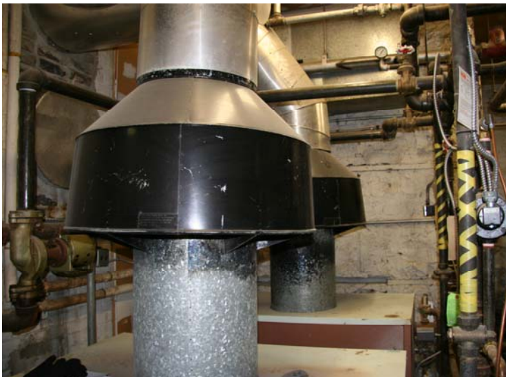
Figure 2.62. Natural gas-fired, hot water radiation system located in the basement of the 1902 section. Image by Natalie Foidart.
