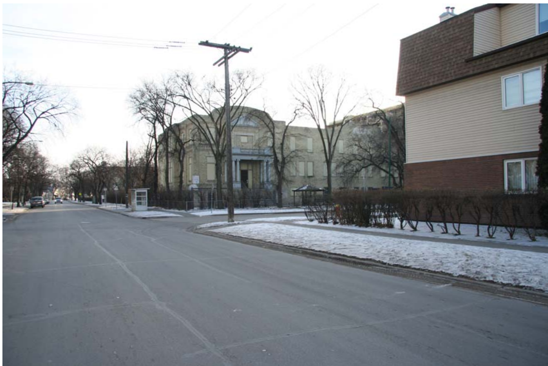
Figure 2.2. View of the north façade of the design investigation building, taken from the far north end of rue Aulneau near its intersection with boulevard Provencher. Image by Natalie Foidart.
