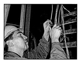
Figure 3-16: Preparing Wires for Splicing
