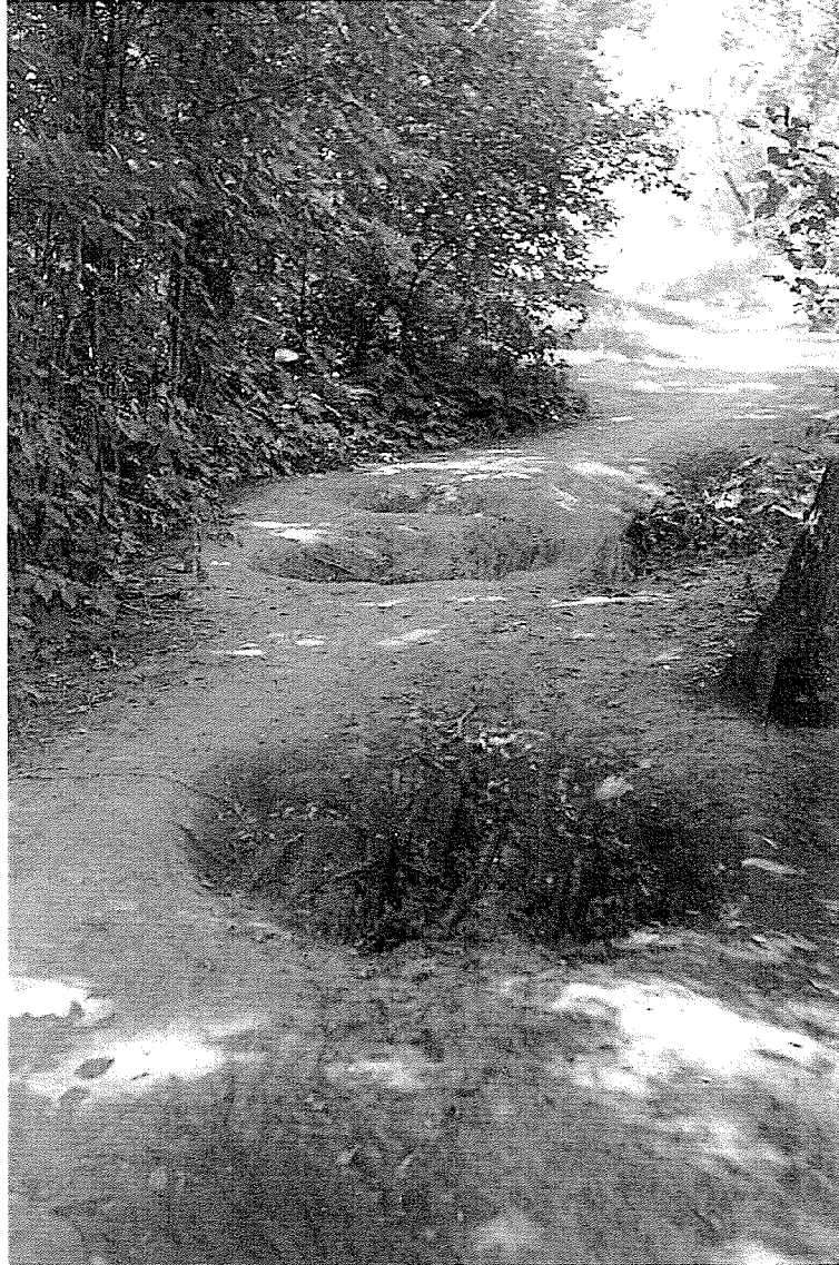
Figure 6.1.5: Severe erosion and pitting along the Assiniboine Park riparian forest trails, immediately west of the Assiniboine Park footbridge (Fabbri & Jurkow 1997).
