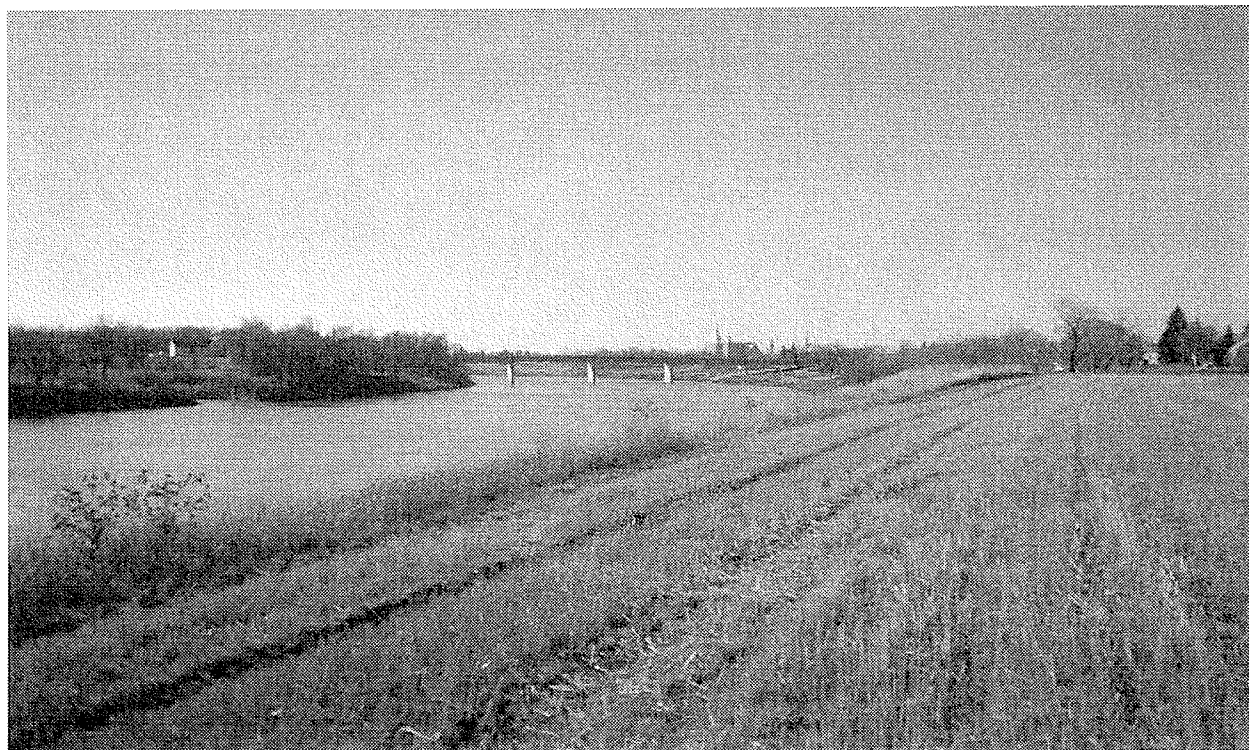
Figure 6.9 – Ste. Agathe bridge, view from north of town
