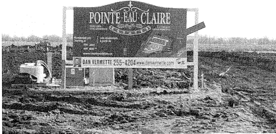
Figure 6.19 – Subdivision sign showing location of new dike
