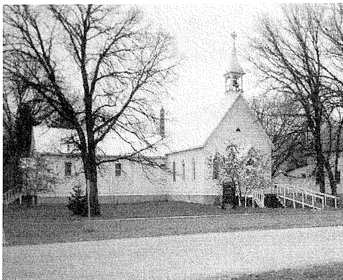
Figure 6.28 – Historic Anglican Church
