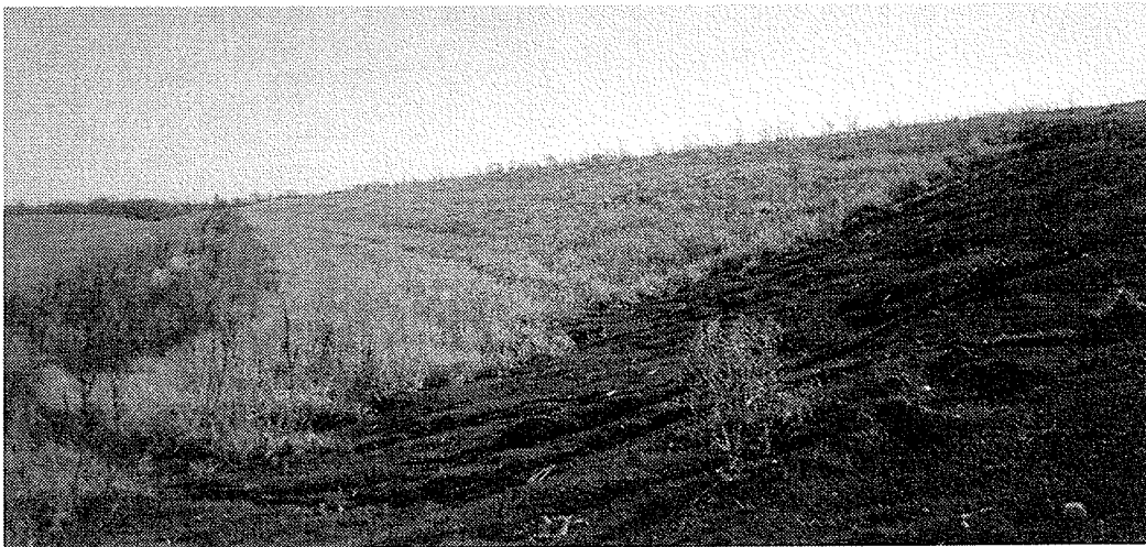
Figure 6.20 – New town dike
