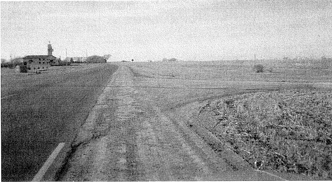
Figure 6.30 – Dike on west side of the Red River
