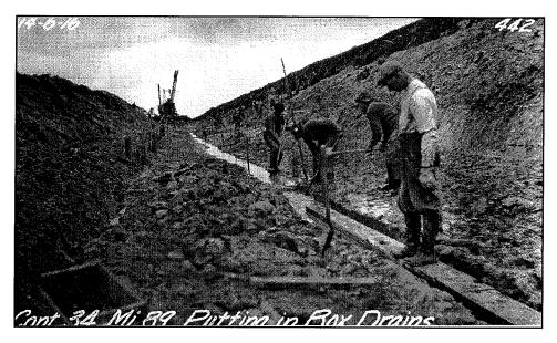
Figure 3-24. Wooden box drains installed just below grade to help control groundwater seepage. (Construction Photograph No. 442)
