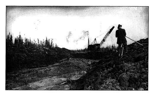
Figure 3-20. Approximately 1.0 to 1.5 metres of base heave in the aqueduct trench, Mile 85.5. Note the spoil banks adjacent to the excavation. (Construction Photograph No. 334)
