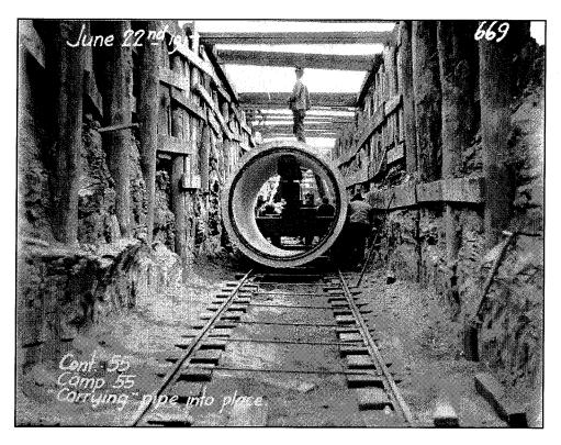
Figure 3-4. Pre-cast pipe segment in shored trench. (Construction Photograph No. 669)
