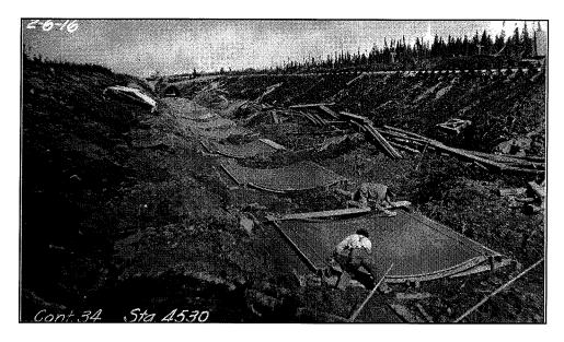
Figure 3-16. Cast-in-place inverts constructed in 4.57 metres lengths. (Construction Photograph No. 418)
