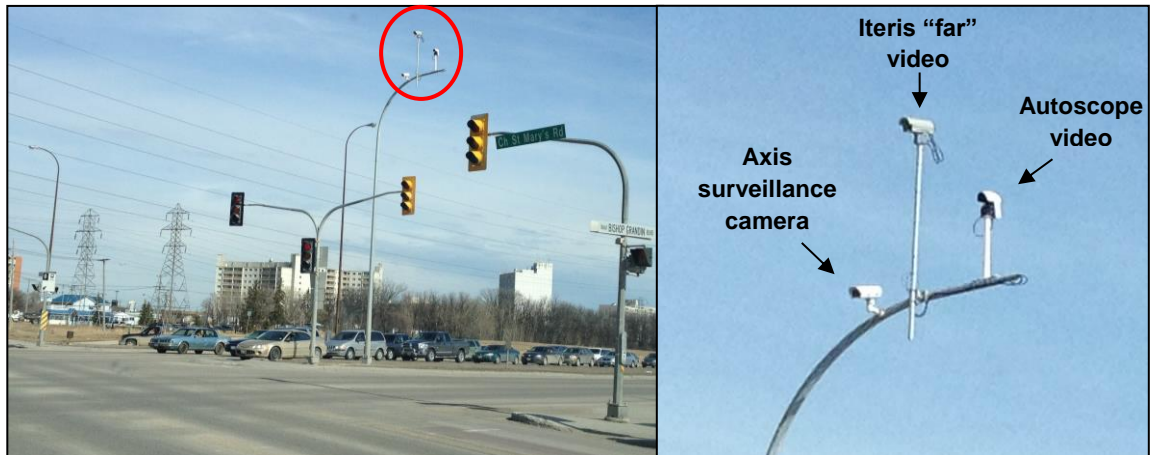
Figure 2: Overhead-mounted video detection sensors ( Iteris far and Autoscope ) and surveillance camera
