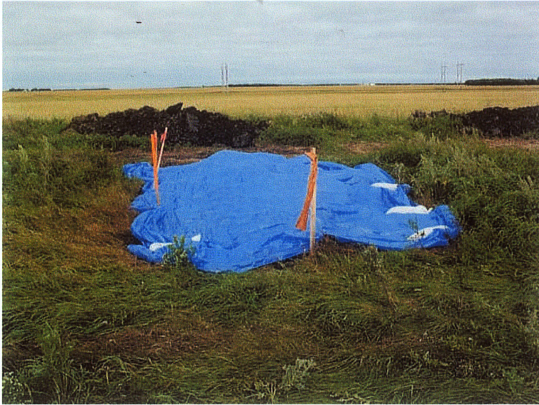
Figure 5: Photo of a completed treatment. The trench has been filled with the mixed product, cages inserted, covered with dirt and tarped.
