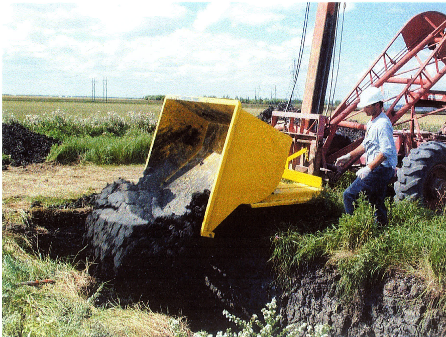
Figure 3: The mixed product being dumped into the trench
