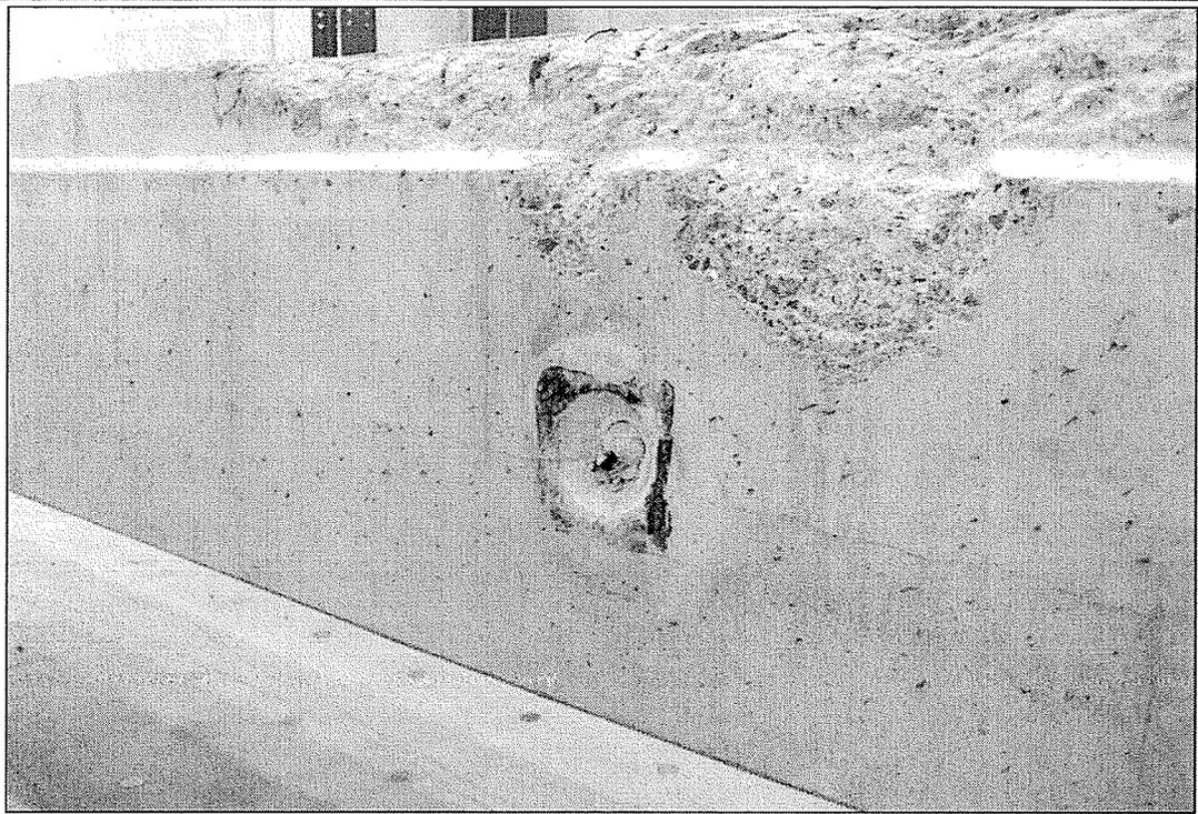
Figure 3-13: Cracking and water leakage stains on the web at the post-tensioning ducts of girder four.
