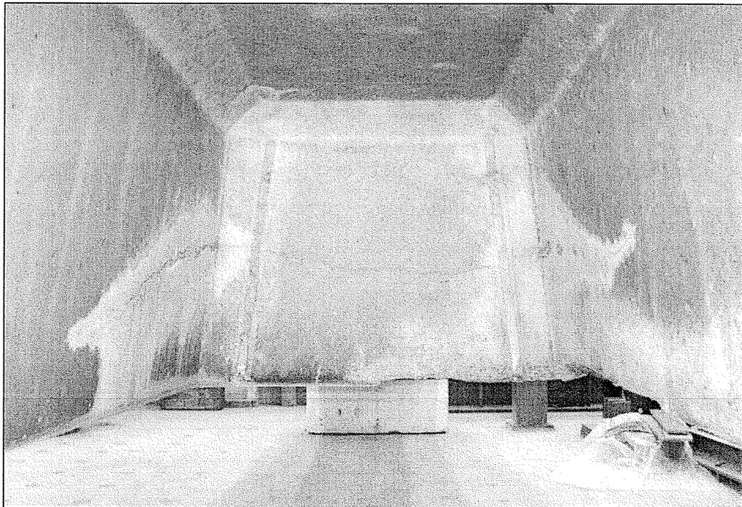
Figure 3-11: Transverse cracking through the diaphragm of girder three.
