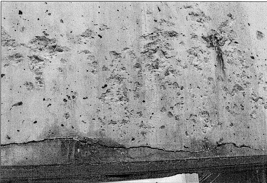
Figure 3-17: Web cracking and delamination, corrosion staining and surface scaling of girder five.
