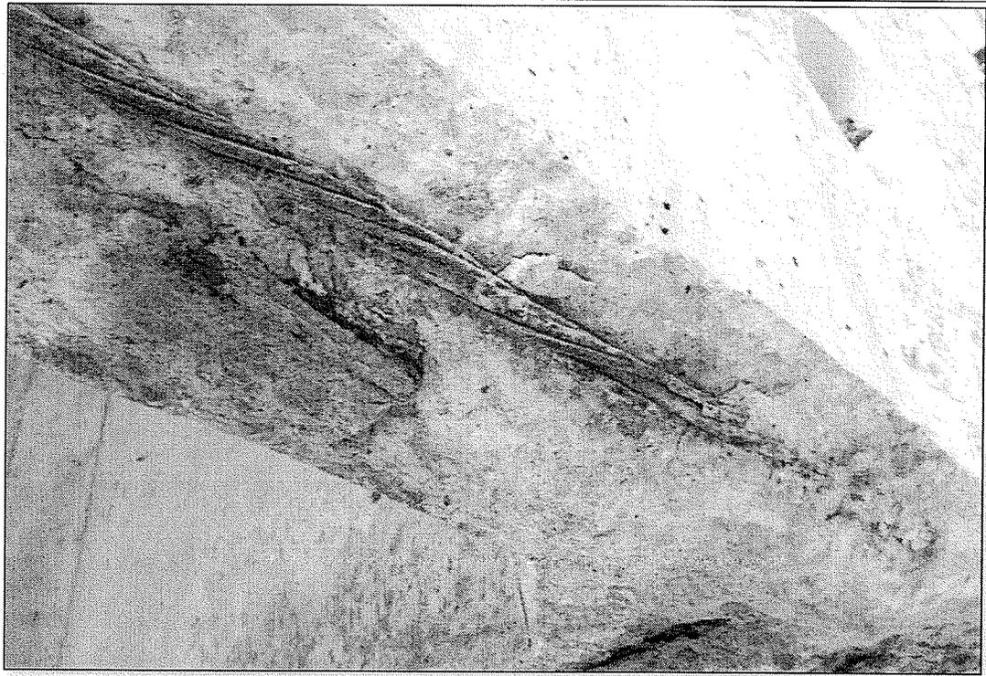
Figure 3-19: Exposed and corroded strands on the web of girder six.
