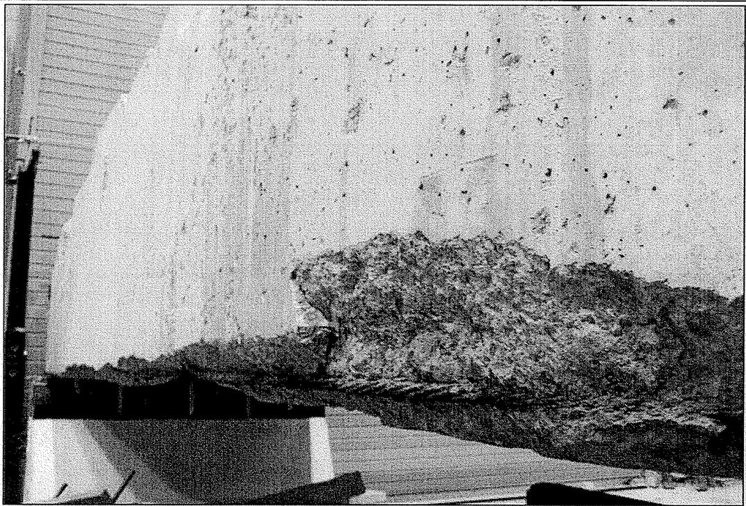
Figure 3-16: Significant concrete loss on the east web near support of girder five.
