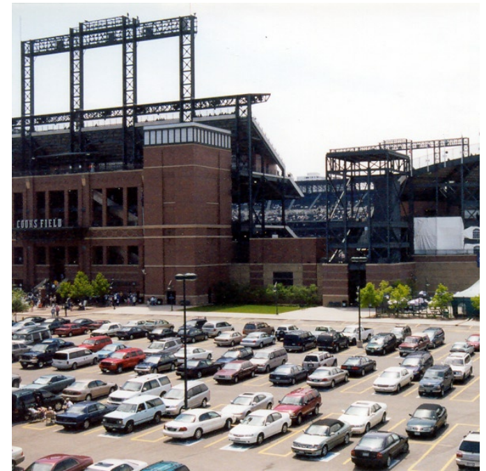
Surface parking behind the ballpark
