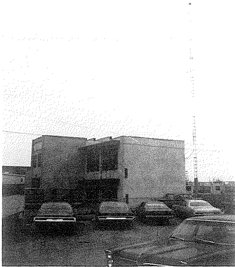
The ITV Centre located at 3195 Portage Avenue, in St. James-Assiniboia. The 100' tower structure supports an all-direction transmitting antenna, local VHF-TV receiving antennae and long wire antennae for short-wave communication.
