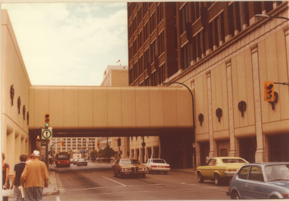
15. Pedestrian Bridge In Downtown
