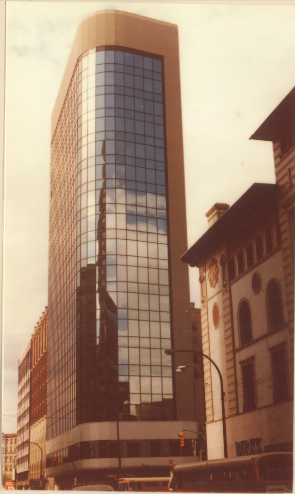
6. First City Trust Building
