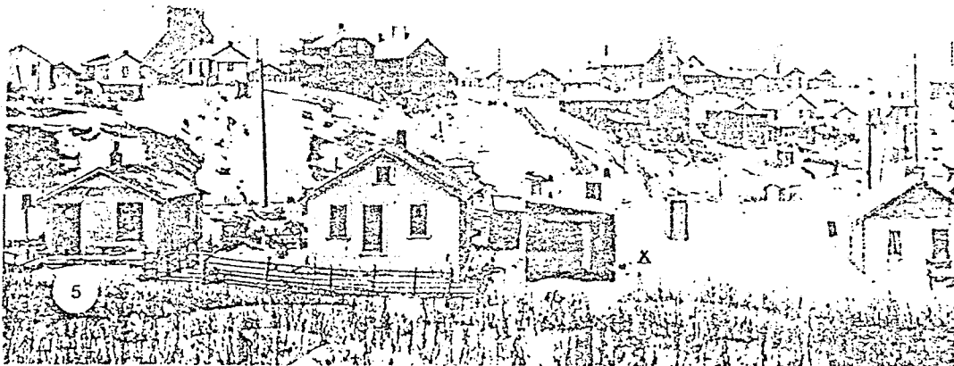
Fig. II. 4. Permanent Development Close To The Mine Shaft
