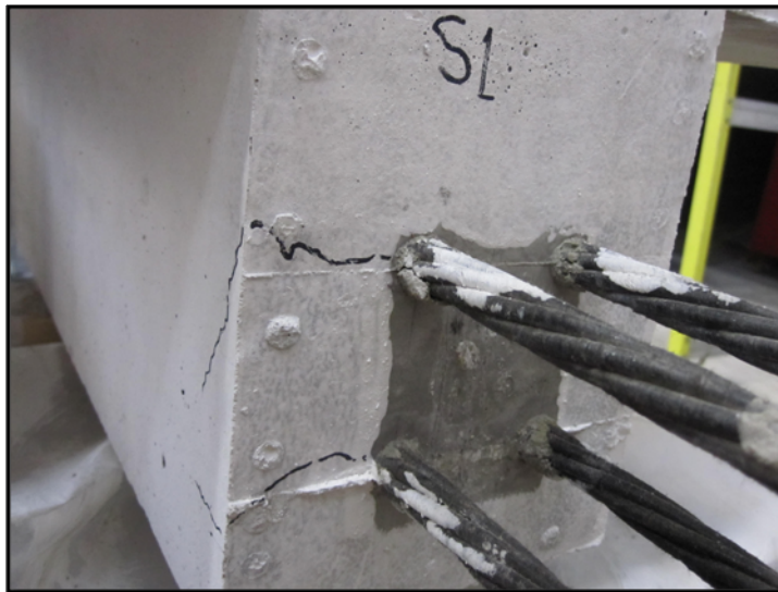
Figure 5- 1: Bursting cracks around the cables for beam S1-2.5
