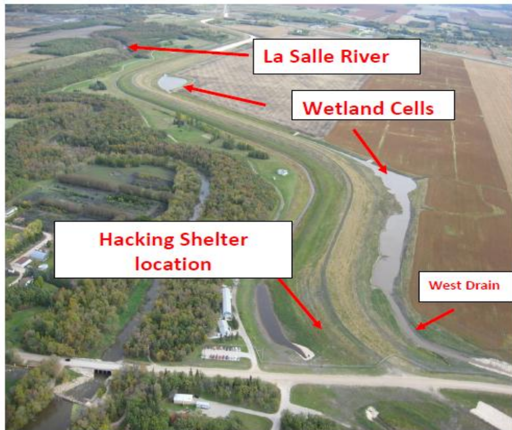
Figure 2.1 - Aerial view of Parkland Mews site (Robert Wheeldon, 2010)
