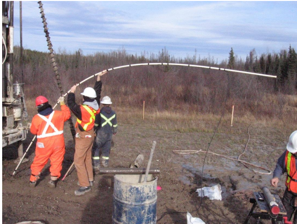
Figure 3.11: Instrument installation into the hole
