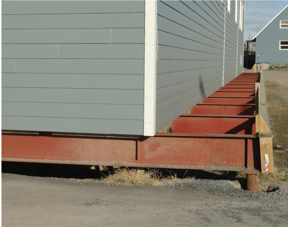
Figure 2.11: Buildings above original ground level, Inuvik, NWT, Canada (photo by author)
