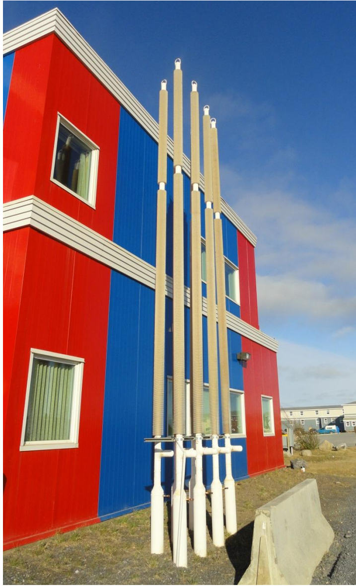
Figure 2.9: Flat Loop Thermosyphon foundations at Inuvik Regional Hospital in Inuvik, NWT, Canada (photo by author)
