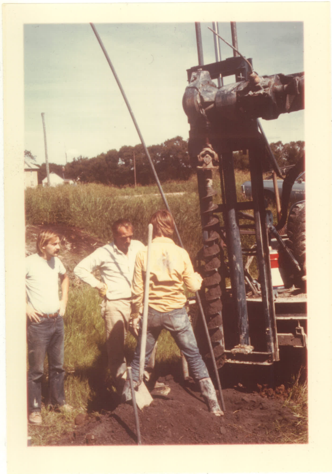
Plate 4 Solid stemmed auger used to install piezometers to depths of 100 feet below ground level. Samples of the different geologic deposits were obtained from the auger.
