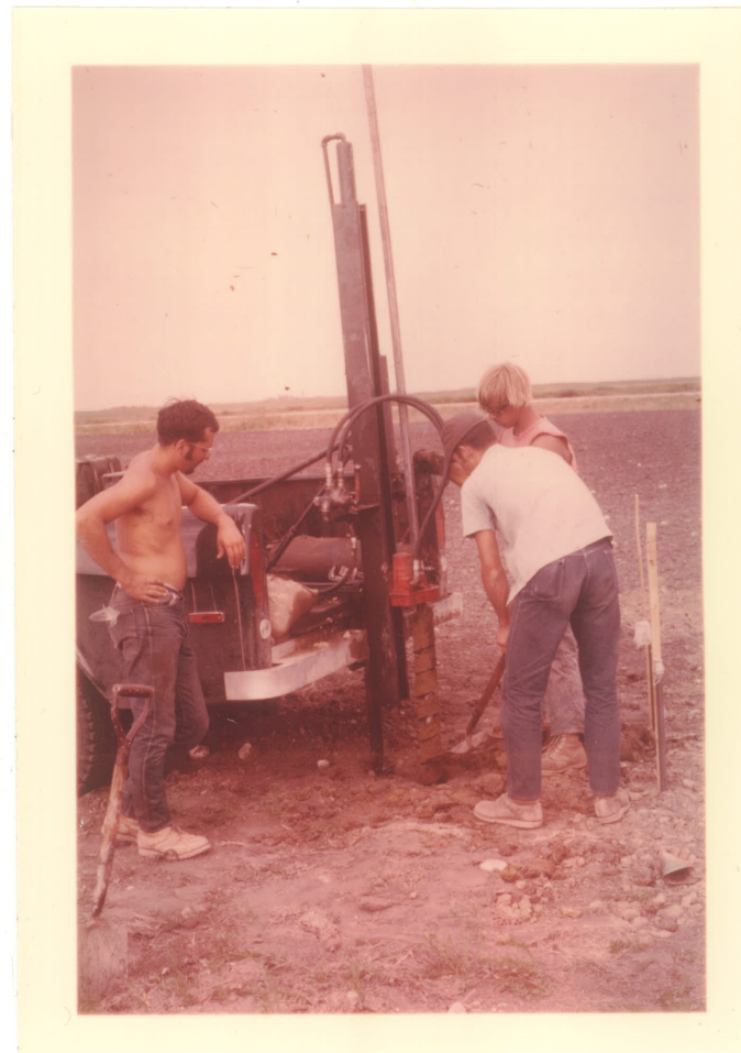
Plate 5 Giddings Drill used to install water table wells and collect soil samples to depths of 10 feet. Soil samples taken directly from auger at intervals of 1 foot.
