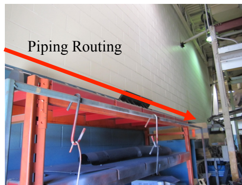
Figure 4: Photograph showing piping placement [3]
