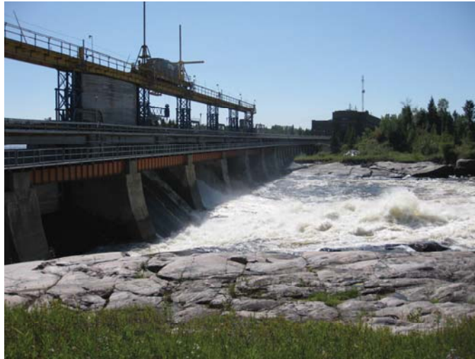
Figure 3.3. The Slave Falls GS spillway, as seen from the downstream side looking south. Photo taken 26 August, 2010, when spillway discharge was approximately 430 \text{ m}^3/\text{s} .
