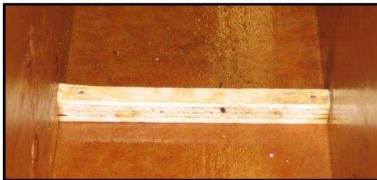
Before Casting [Inside Formwork]
