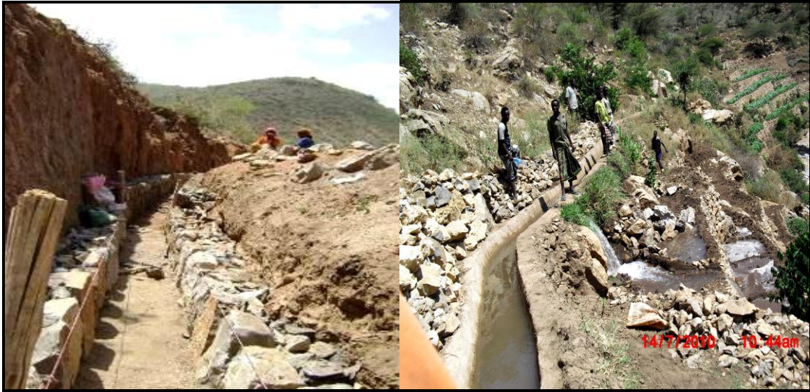
Plate 16. Small-scale Irrigation Canal (during construction and after)
