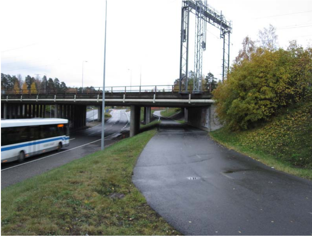
Figure 22: A pathway parallels a high-volume roadway. Photo credit: Author
