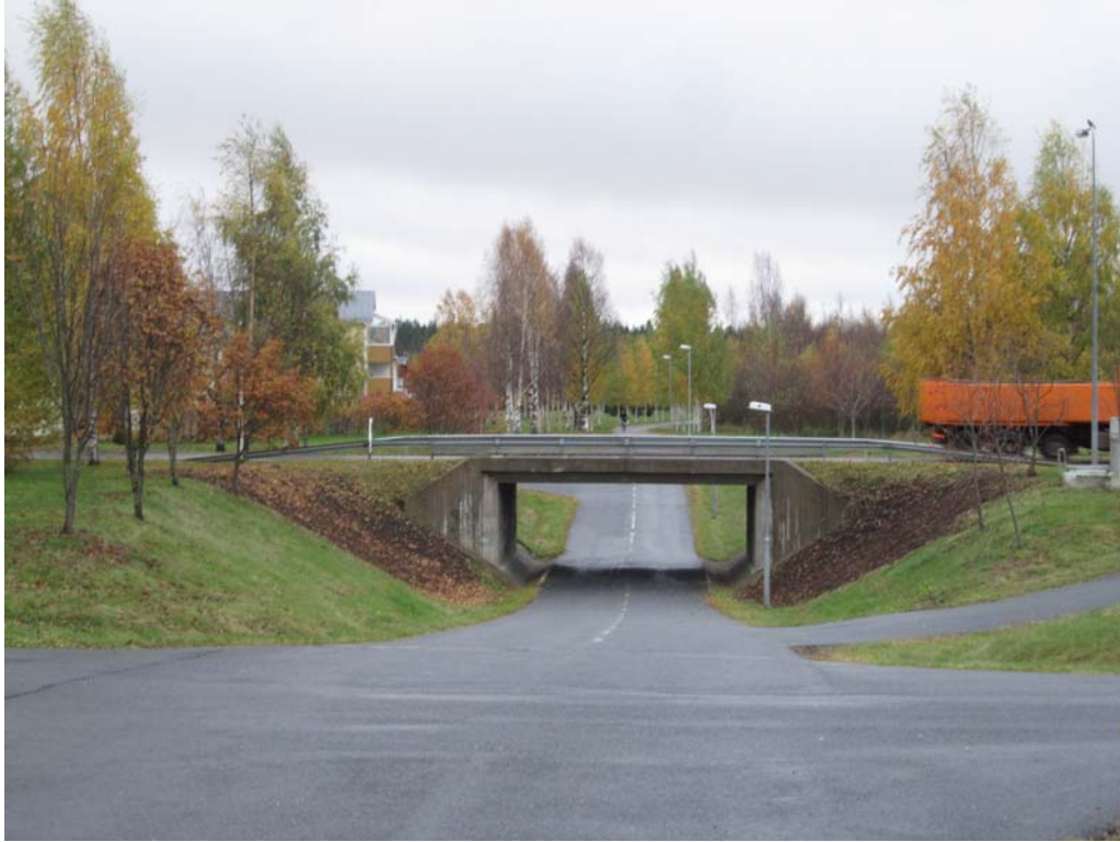
Figure 18: Grade separation in Oulu. Pathways converge, pass underneath a roadway. Photo credit: Author
