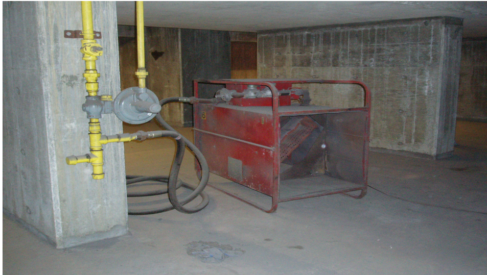
Figure 41: Direct-fired natural gas heater
