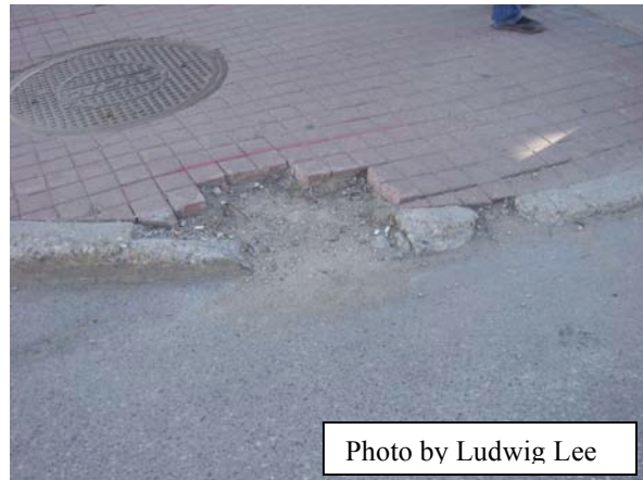
Fig 5: Existing sidewalk and curb corners are in poor condition and pose tripping hazards for pedestrians.
