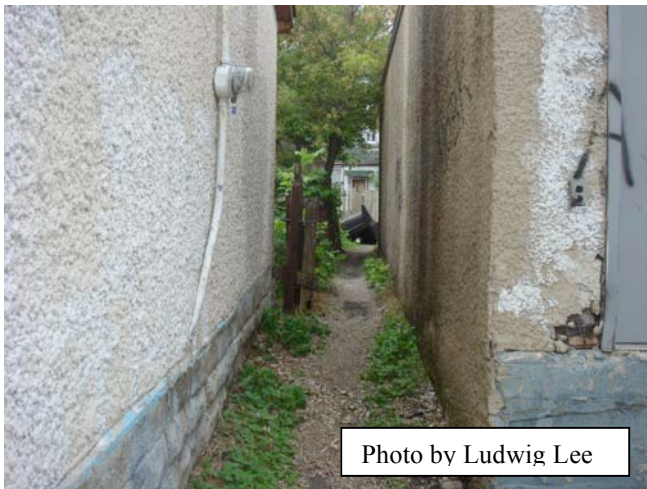
Fig 6: Example of a cut-through on private property between two buildings.
