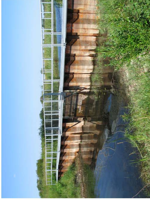
Figure 3-3: Summerberry water control structures. Top left: 35HI weir, viewed from the wetland. Top right: 37C weir, viewed from the Saskatchewan River, releasing water. Bottom left: 14R weir, viewed from the back channel. Bottom right: 32C gated culvert control structure. Other control wetlands had similar gated culvert controls, which were not operated during 2007 and 2008. Photography by Dale Wrubleski.
