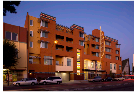
Figure 10. Exterior of Seven Directions. Image courtesy of Pyatok Architects.
