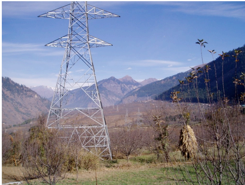
Plate 7. Transmission Line crossing agricultural land (J. Gardener, 2008)
