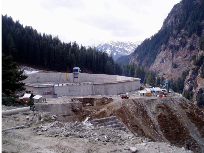
Plate 4. AD project holding tank being built in Hampta Valley (J. Gardener, 2008)
