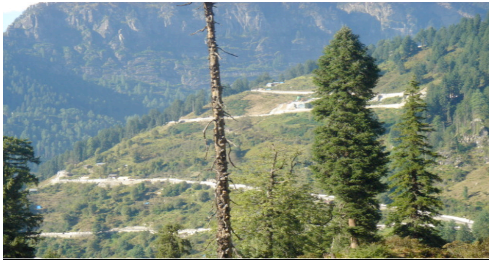
Plate 4: Access road created at the project site (V.Lozecznik, 2008)
