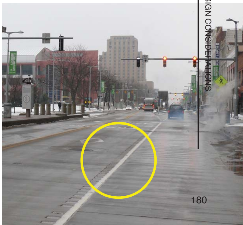
Figure 65. Euclid Corridor rumble strip lane separation.
