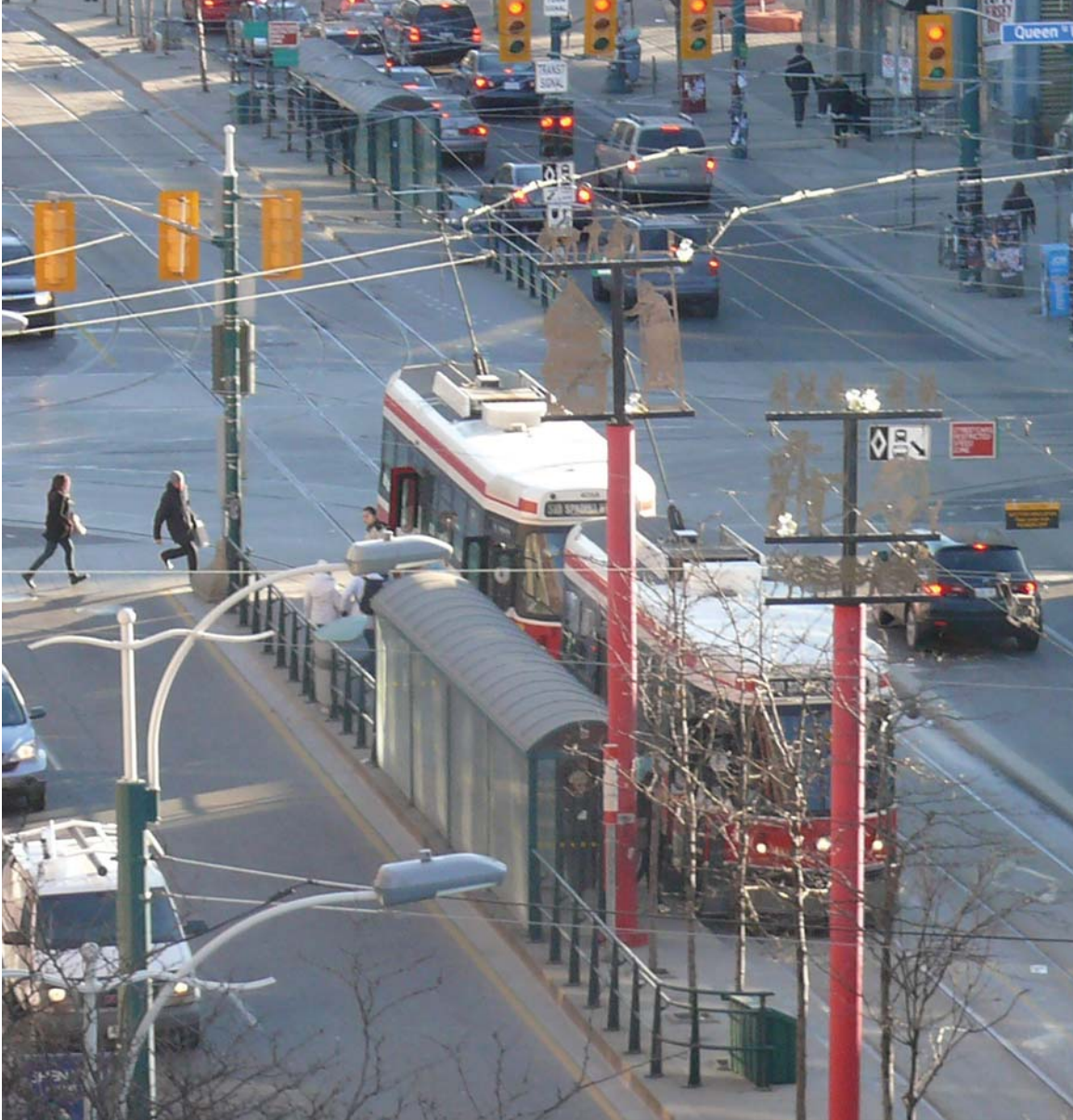
Figure 75. Spadina station corals riders to signalized intersections.
