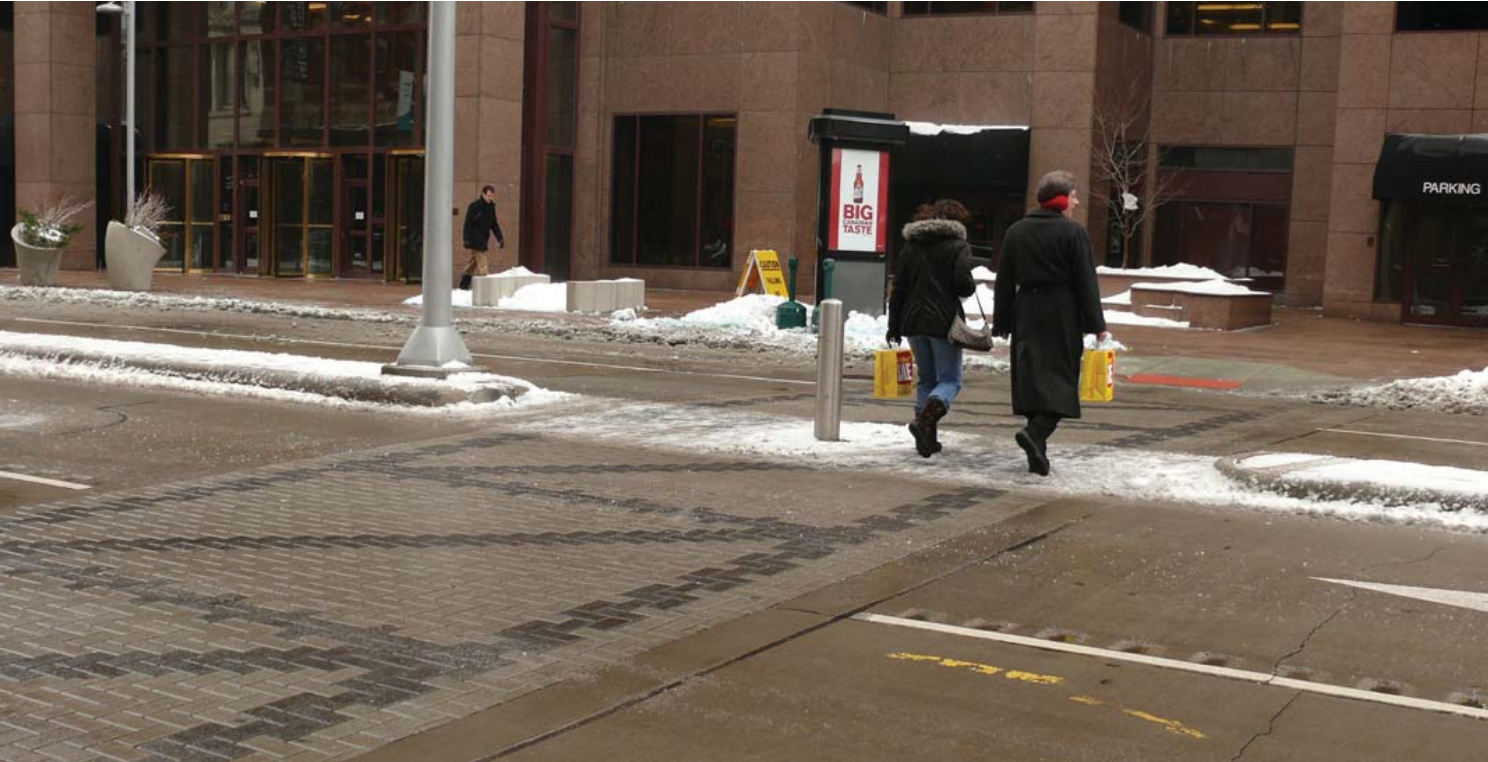
Figure 74. Euclid Avenue, mid block crosswalk, “Z” pattern promotes visibility for drivers and safety for pedestrians.
