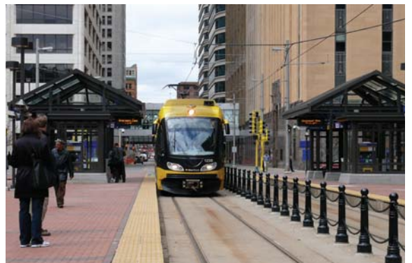
Figure 70. Fenced track separation, Hiawatha Line, Minneapolis.
