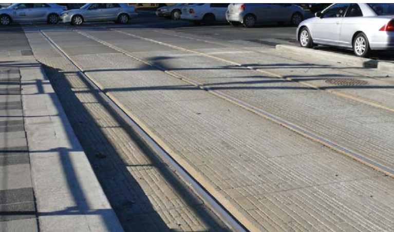
Figure 71. Stamped concrete, St. Clair streetcar Line, Toronto.
