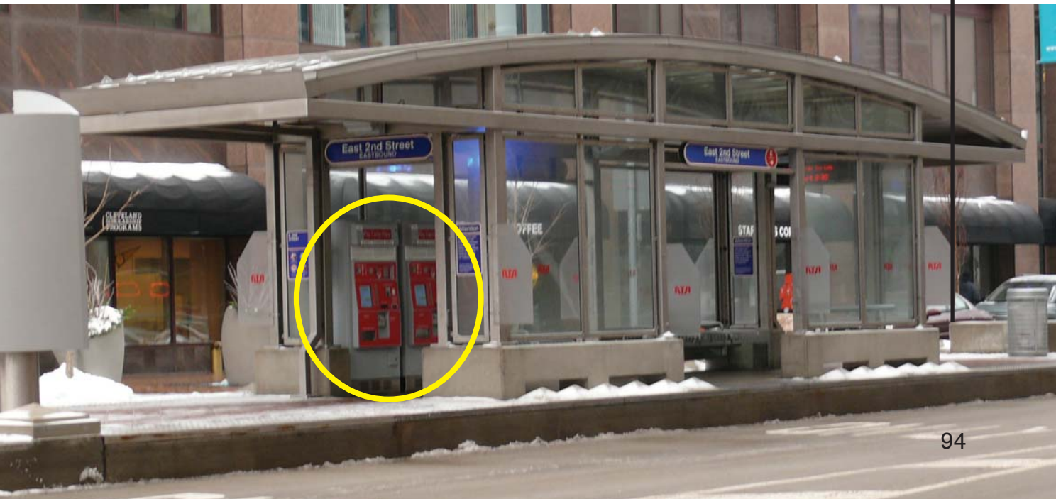
Figure 41. Modern station design and automated ticket machine. Euclid Corridor, Cleveland.
