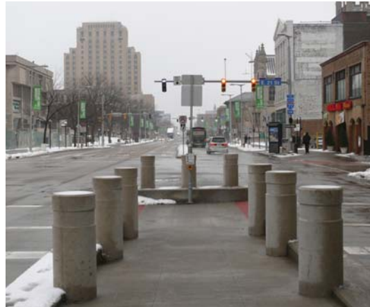
Figure 77. Bollards at a Euclid Corridor station corral riders to signalized intersections.
