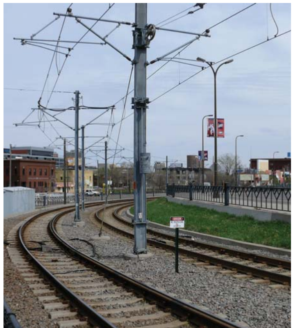
Figure 69. Hiawatha Line ballasted track.
