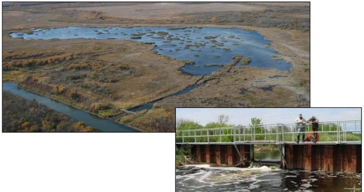
Figure 1.9- Example of water control structure placement and design (inset) within wetland 14R in the Summerberry Marsh Complex, Manitoba.
