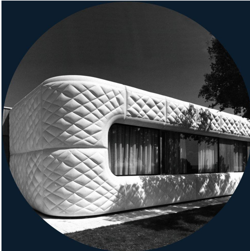
Figure 4: Prefabricated cladding for a house formed with flexible formwork and white cement by Miguel Fisac (Arnardóttir and Merina 2008)
