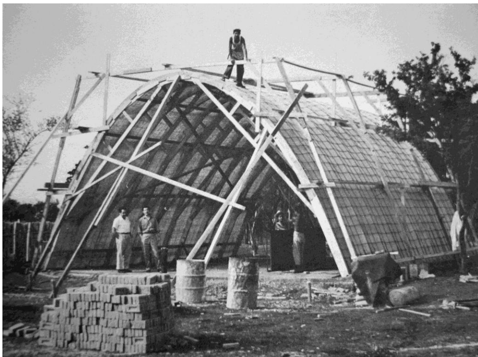
Figure 3: Vault for a rural school in Tamaulipas, Mexico, designed by Felix Candela. (Faber 1963)
