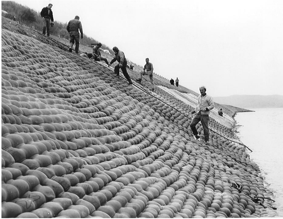
Figure 5: River bank stabilization bags (Fabriform) installed in 1967 on the Allegheny Reservoir, New York ( www.fabriform1.com 2009)
