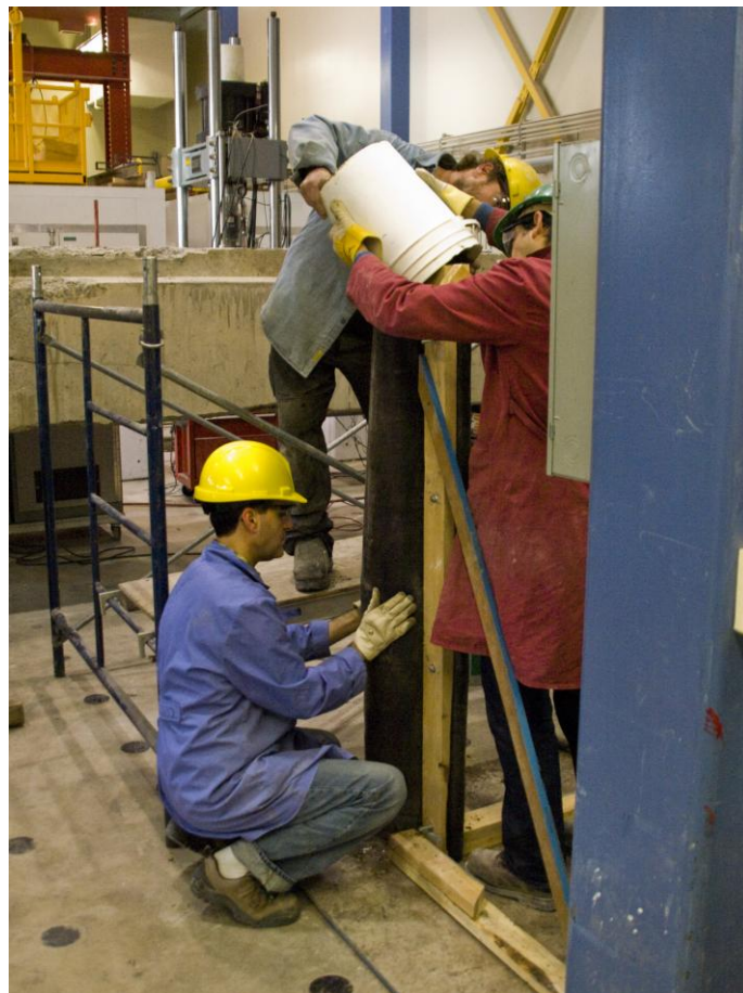
Figure 47: casting of column in fabric formwork
