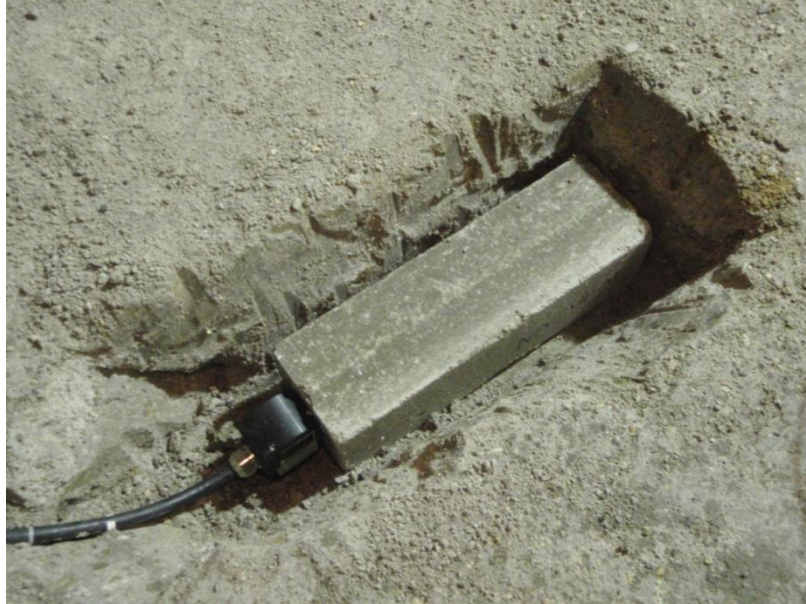
Figure 5.57: Time domain reflectometry probe installation prior to backfilling (AECL stock photograph)
