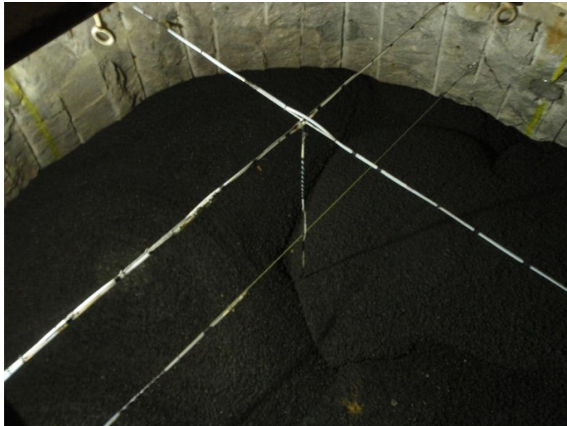
Figure 4.17: Partially completed pour of the upper concrete component showing instrument support cables (AECL stock photograph)
