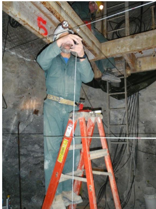
Figure 5.63: Installing a vertical instrument support cable in the upper concrete component (AECL stock photograph)
