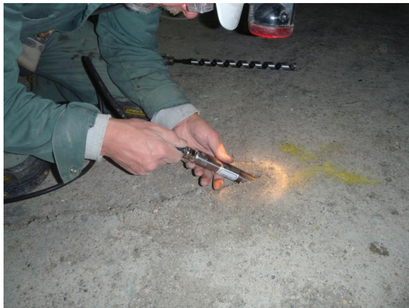
Figure 5.47: Installing a piezometer in the bentonite sand component (AECL stock photograph)
