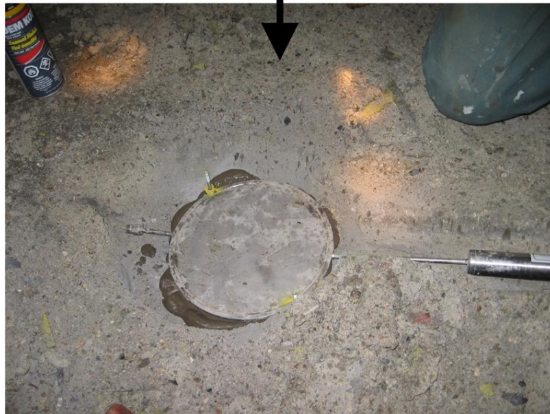
Figure 5.48: Installation of a total pressure cell at the lower clay-concrete interface (AECL stock photographs)
