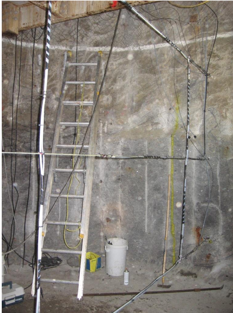
Figure 5.65: Installation of deformation sensors in the upper concrete component, looking south (AECL stock photograph)
