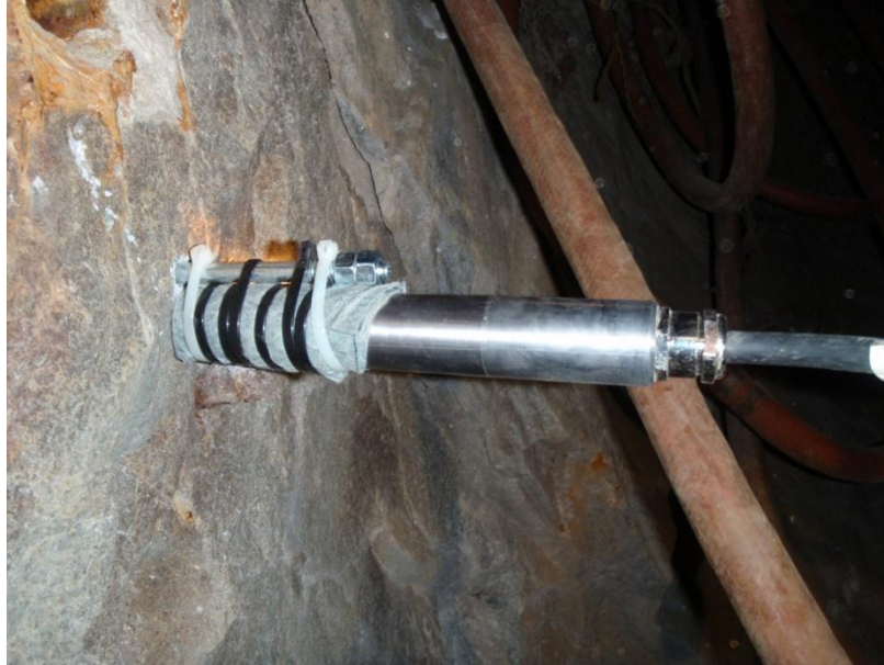
Figure 5.67: Installation of a vibrating wire piezometer at the upper concrete-rock interface (AECL stock photograph)
