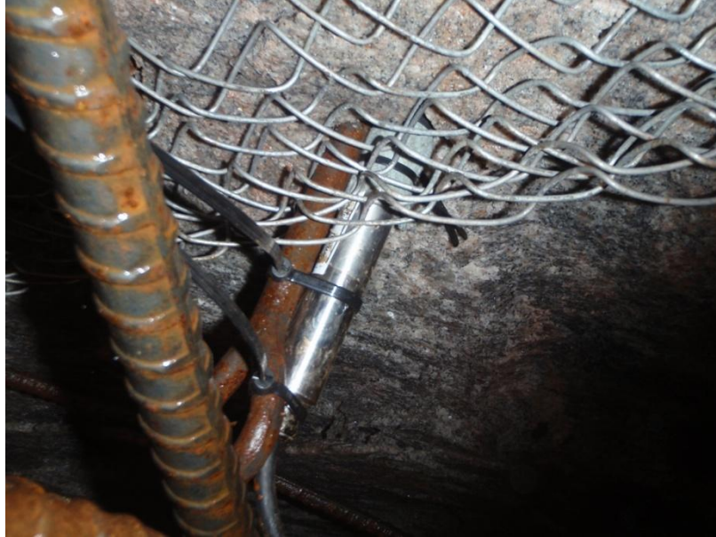
Figure 5.44: Installation of a vibrating wire piezometer on an I-bolt at the lower concrete-rock interface (AECL stock photograph)
