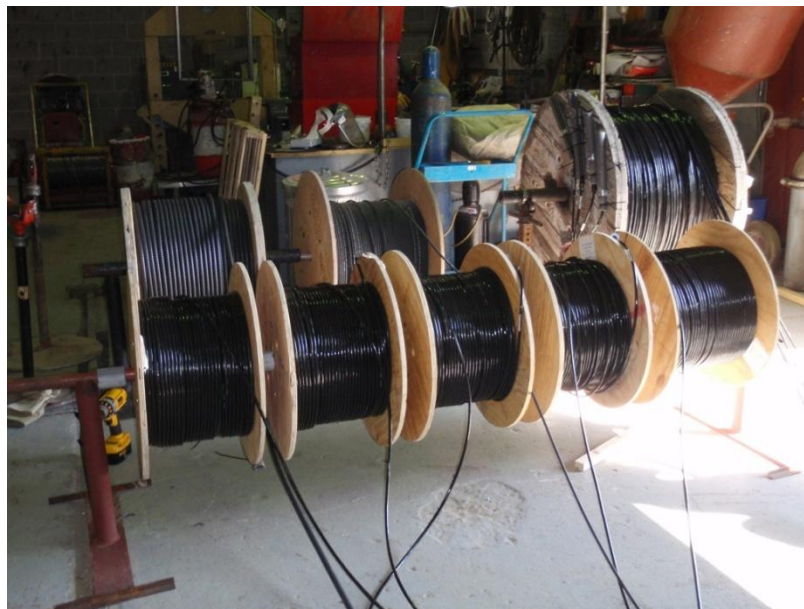
Figure 5.28: Cable bundles on cable stands ready to be lowered down shaft (AECL stock photograph)
