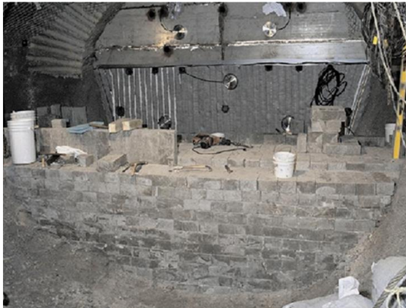
Figure 2.18: Pre-compacted block construction of the TSX clay bulkhead (Chandler, et al. 2002)
