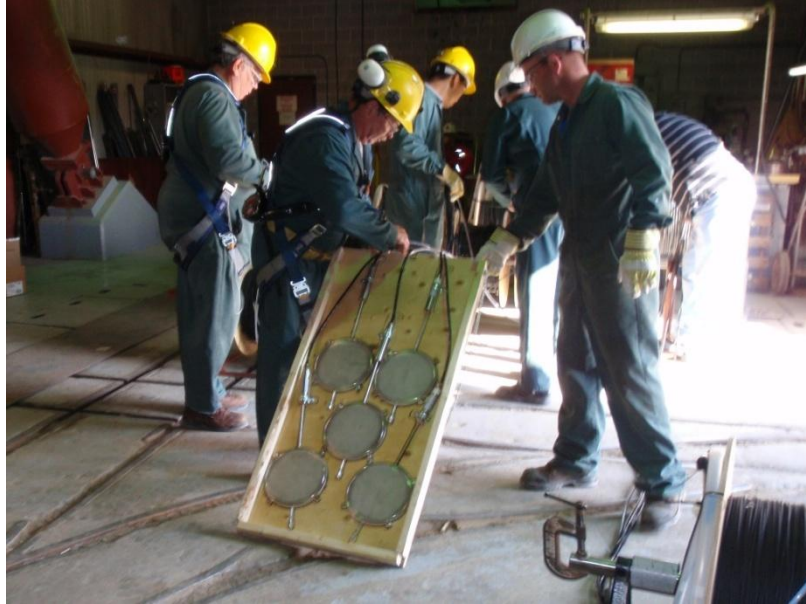
Figure 5.30: Plywood protection and support for total pressure cells (AECL stock photograph)
