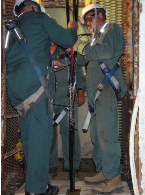
Figure 5.32: Attaching cables to the messenger wire (AECL stock photograph)
