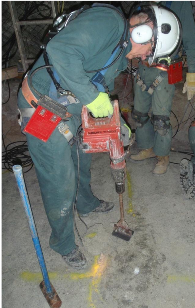
Figure 5.53: Backfilling and compaction after installing a total pressure cell in the bentonite-sand component (AECL stock photograph)
