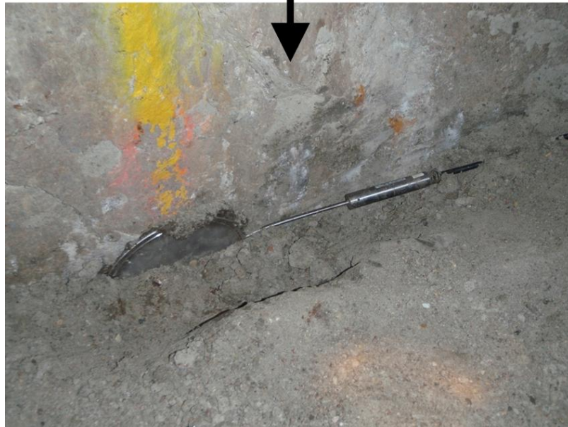
Figure 5.51: Installation of a horizontal total pressure cell at the clay-rock interface (AECL stock photographs)
