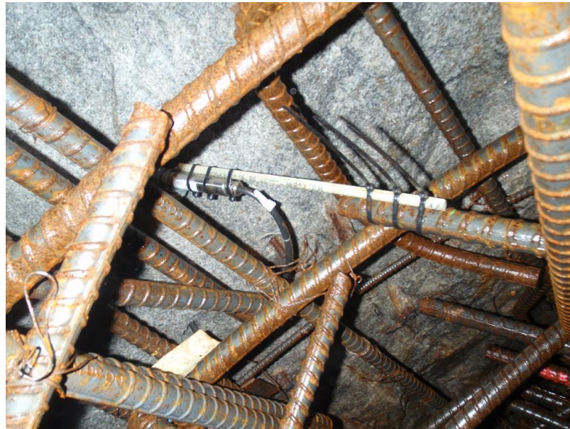
Figure 5.43: Installation of a vibrating wire piezometer on rebar at the lower concrete-rock interface (AECL stock photograph)
