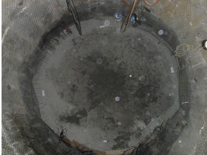
Figure 4.16: Top view of the completed bentonite-sand component (AECL stock photograph)
