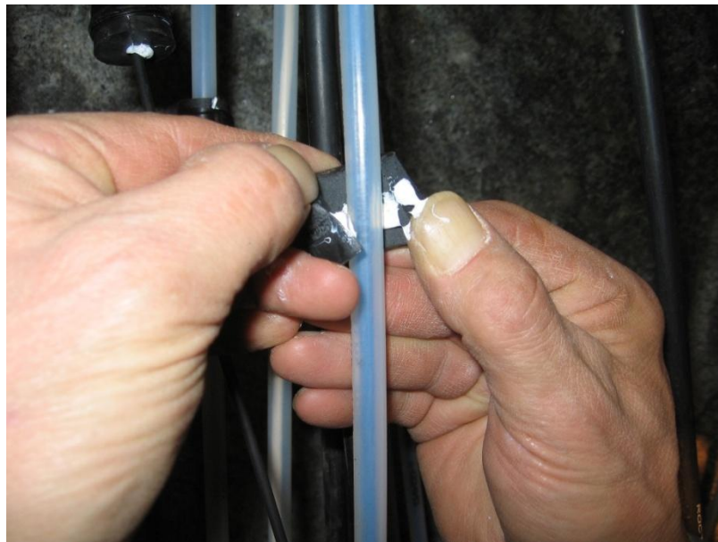
Figure 5.76: Installing an instrument cable water stop in the upper concrete component (AECL stock photograph)
