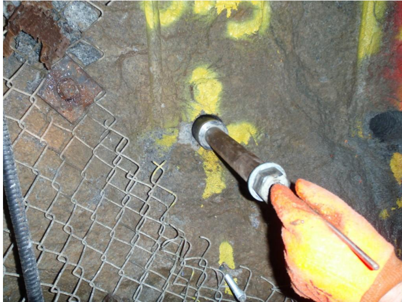
Figure 5.59: Inserting a mechanical packer into a horizontal borehole (AECL stock photograph)
