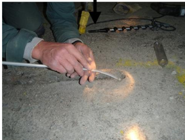
Figure 5.54: Installation of a thermocouple psychrometer (AECL stock photographs)
