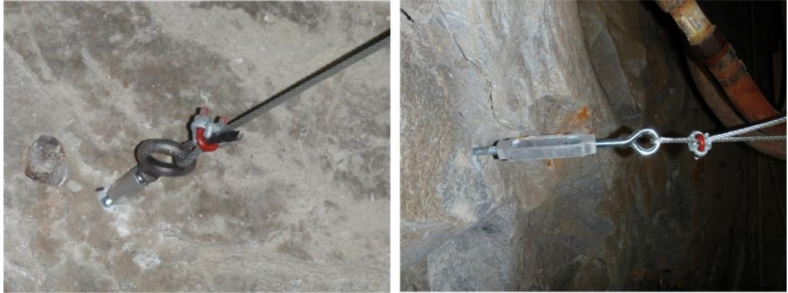
Figure 5.62: Instrument support cable anchors in the upper concrete component, I-bolt (Left) and turnbuckle (right) (AECL stock photographs)
