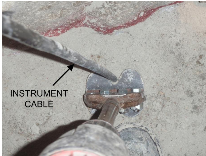
Figure 4.14: Impact hammer compaction foot used near instrument cables (AECL stock photograph)
