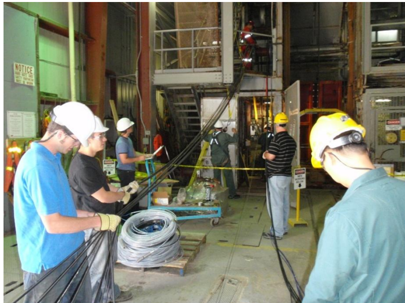
Figure 5.31: Manually reeling out cables during lowering (AECL stock photograph)
