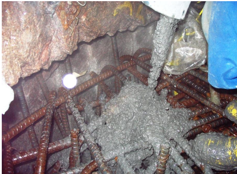
Figure 4.9: Pouring concrete using the flexible rubber chute (AECL stock photograph)
