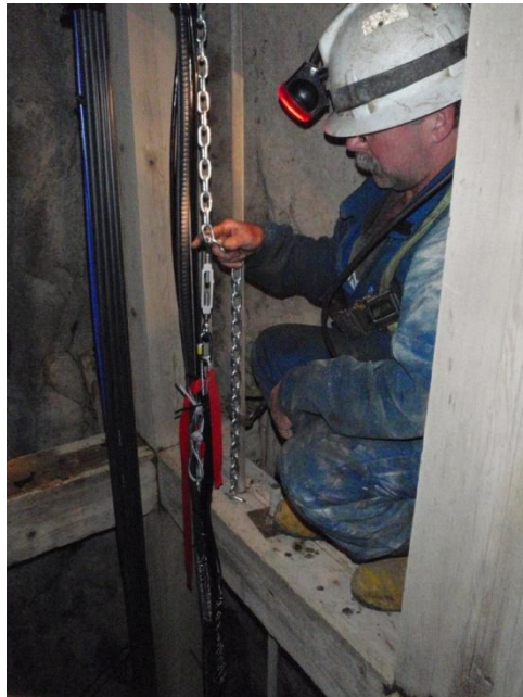
Figure 5.33: Anchoring messenger wire to shaft timbers (AECL stock photograph)
