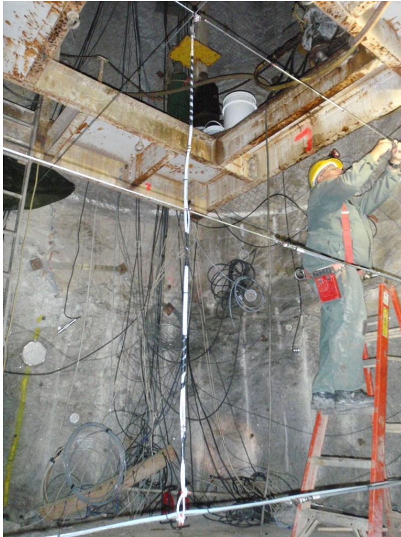
Figure 5.61: Installing instruments on support cables in the upper concrete component (AECL stock photograph)
