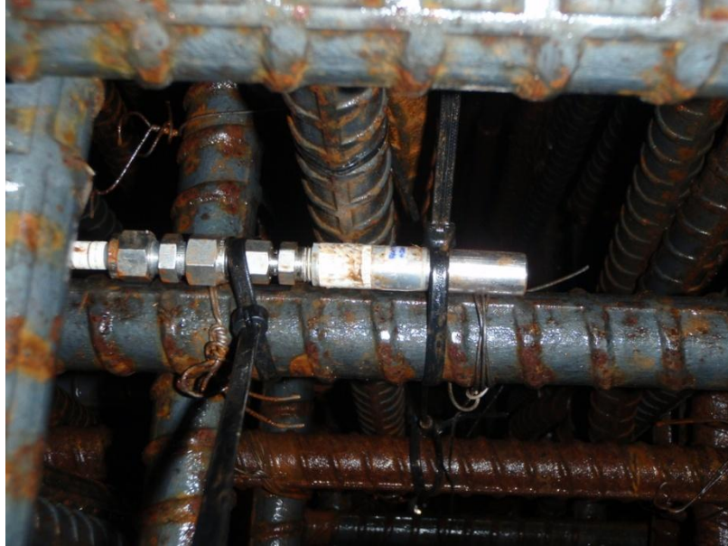
Figure 5.38: Thermocouple (Ct05) installed on the lower concrete component rebar (AECL stock photograph)
