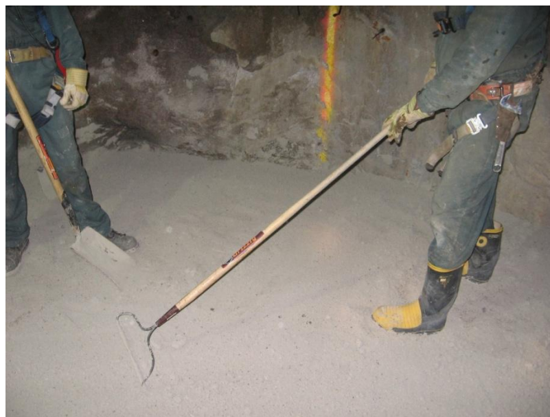
Figure 4.11: Spreading and leveling bentonite-sand material (AECL stock photograph)
