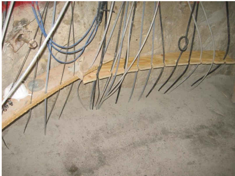
Figure 5.45: Instrument cable separation in the bentonite-sand component (AECL stock photograph)
