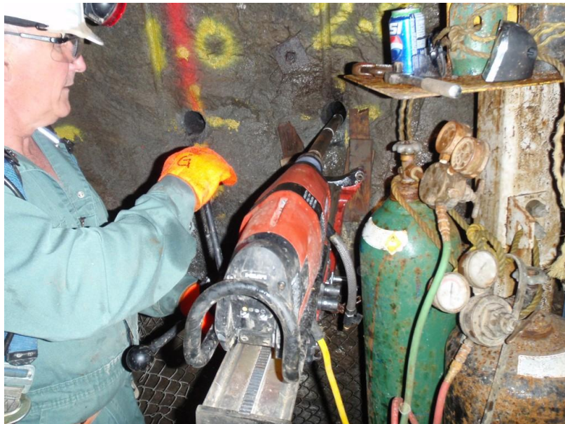
Figure 5.58: Drilling horizontal boreholes for mechanical packers in adjacent rock (AECL stock photograph)
