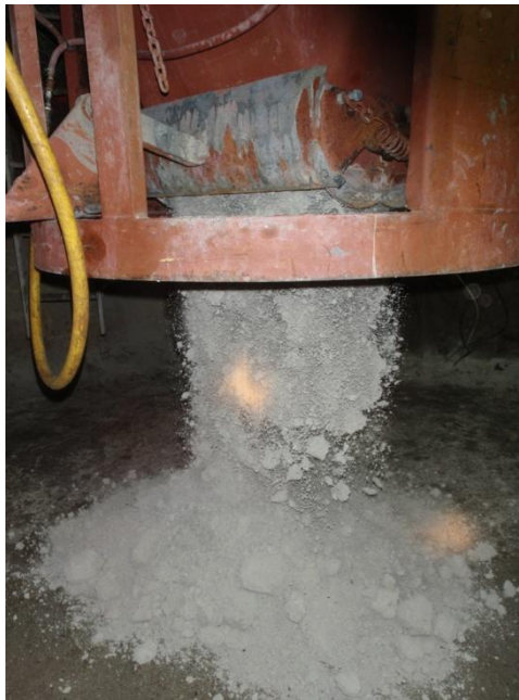
Figure 4.10: Dumping a load of bentonite-sand material (AECL stock photograph)
