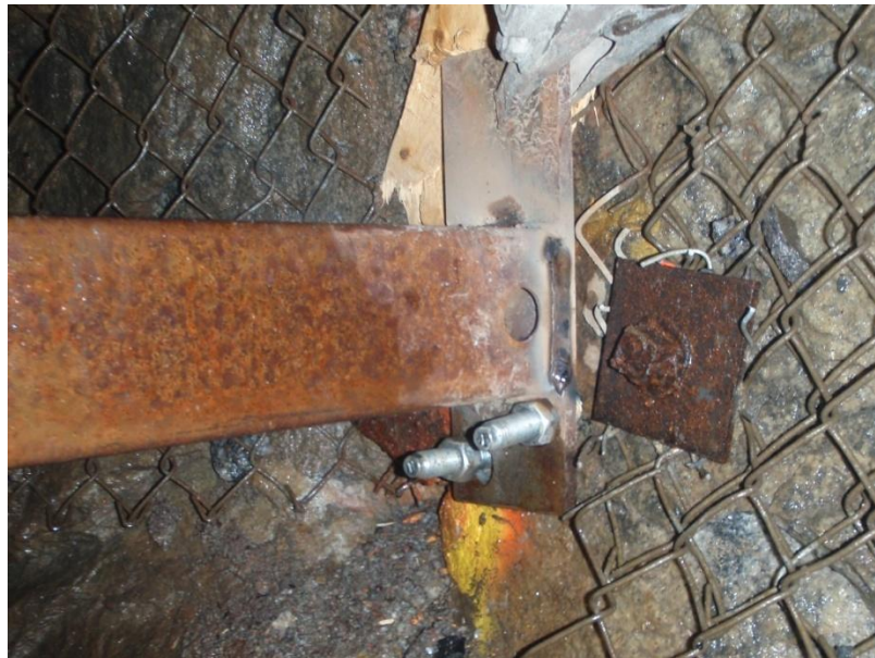
Figure 5.72: Fibre optic displacement transducer mounting beam anchor (AECL stock photograph)
