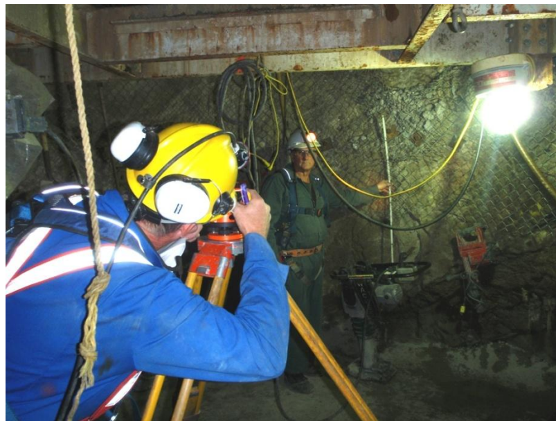
Figure 4.15: Surveying elevation reference lines during bentonite-sand construction (AECL stock photograph)
