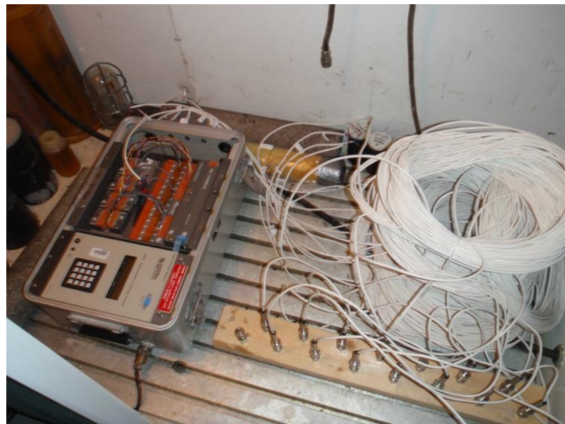
Figure 5.17: CR7X datalogger and psychrometers in environmental chamber (AECL stock photograph)
