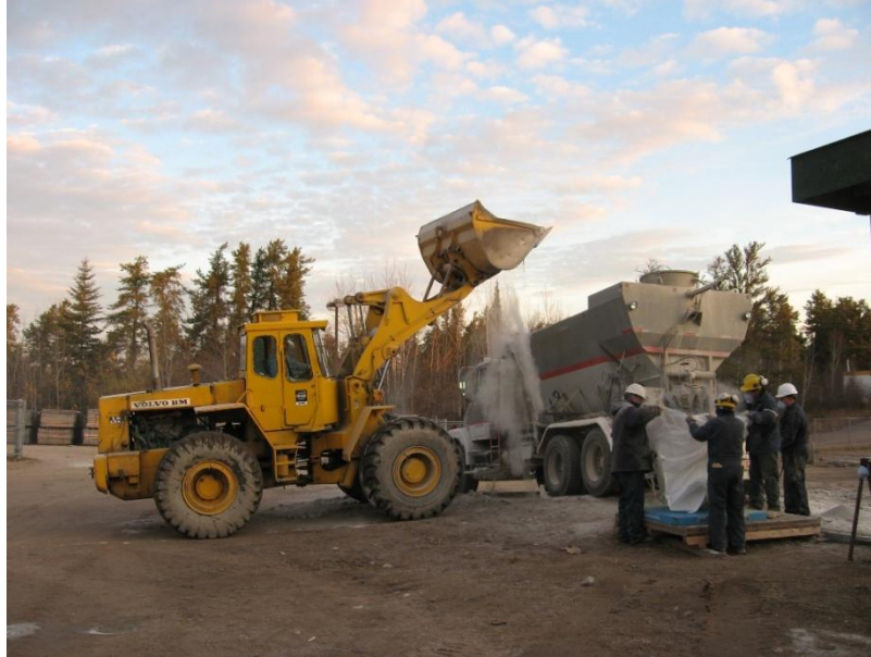
Figure 4.6: Loading the batching truck used to mix bentonite-sand material (AECL stock photograph)
