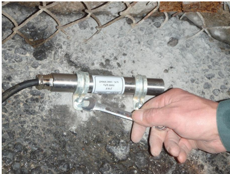
Figure 5.68: Installation of a vibrating wire piezometer on the top surface of the upper concrete component (AECL stock photograph)
