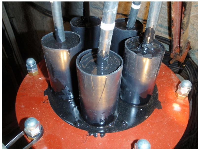
Figure 5.82: Potting the TDR caisson connectors (AECL stock photograph)
