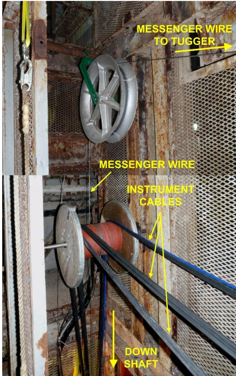
Figure 5.29: Shiv wheel (top) and cable guide (bottom) used to lower shaft cabling (stitched photograph) (AECL stock photographs)
