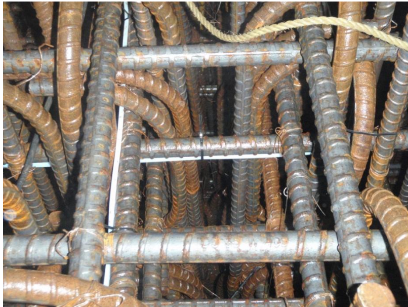
Figure 5.39: Two horizontal deformation sensors installed on the bottom concrete component rebar (AECL stock photograph)
