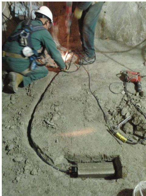
Figure 5.56: Installation of a time domain reflectometry probe (AECL stock photograph)
