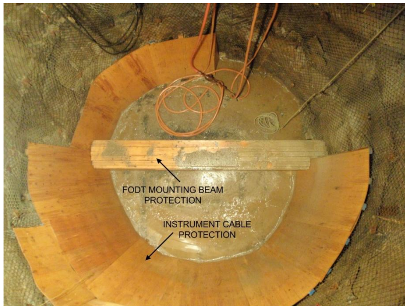
Figure 5.34: Plywood cable protection at the top of the shaft seal (AECL stock photograph)
