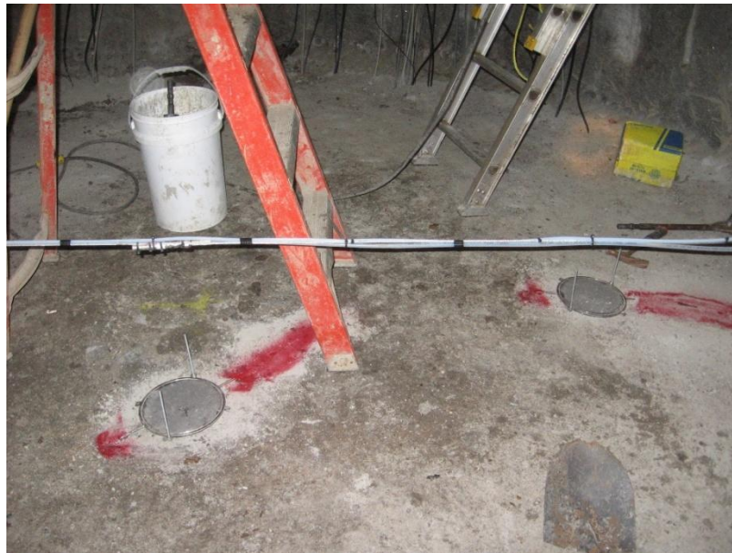
Figure 5.50: Two total pressure cells installed at the upper clay-concrete interface (AECL stock photograph)
