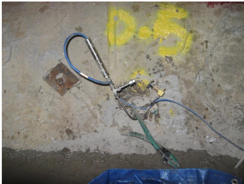
Figure 5.60: Final installation of a mechanical packer with vibrating wire piezometer attached (AECL stock photograph)
