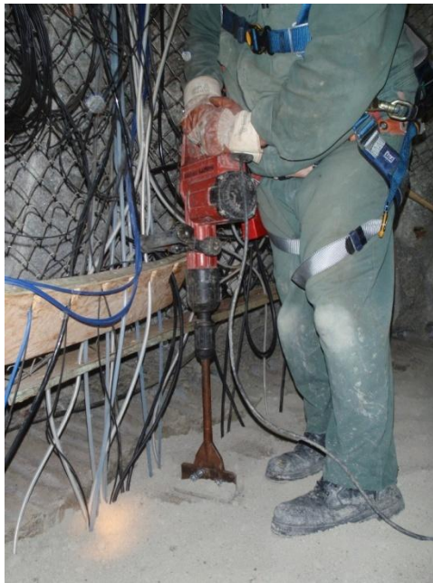
Figure 4.13: Hilti impact hammer used for compaction (AECL stock photograph)
