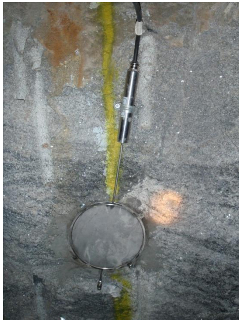
Figure 5.70: Installation of a vibrating wire total pressure cell at the upper concrete-rock interface (AECL stock photograph)
