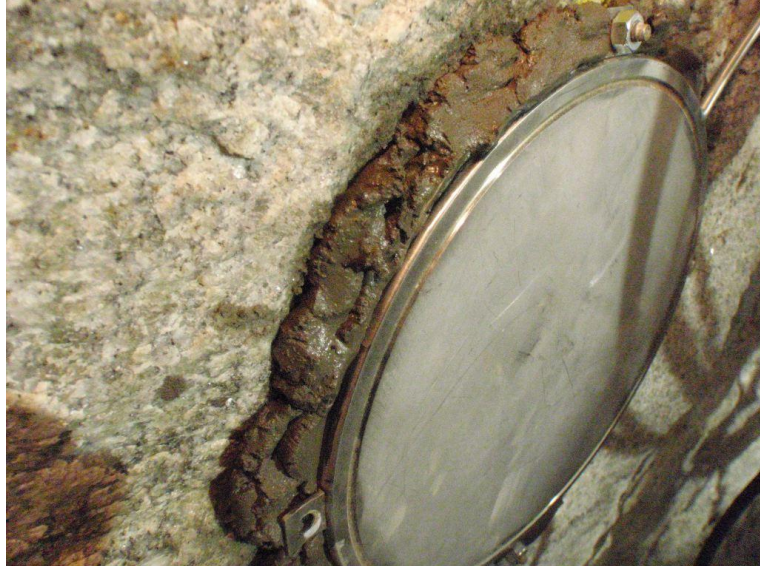
Figure 5.69: Hydraulic cement placed behind the sensing pad of a total pressure cell at the upper concrete-rock interface (AECL stock photograph)
