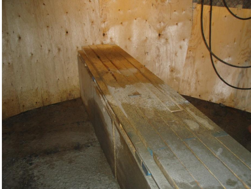
Figure 5.74: Wooden box covering the fibre optic displacement transducer mounting beam (AECL stock photograph)
