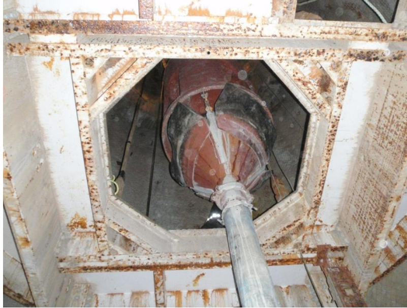
Figure 4.8: Lowering the concrete bucket with flexible rubber chute through the Galloway stage (AECL stock photograph)
