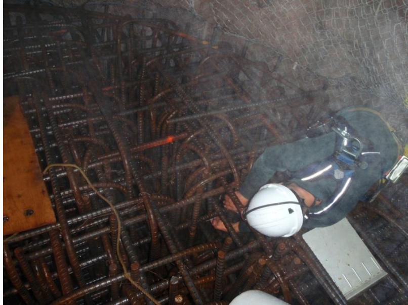
Figure 5.36: Difficulty when installing instruments in the lower concrete rebar (AECL stock photograph)
