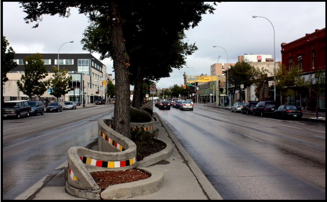
Figure 41. Main Street looking north from Alexander Avenue, 2009. The Edge Gallery and Mitchell Fabrics can be seen on the right (building with green awning), and the Winnipeg Regional Health Authority building can be seen on the left.
