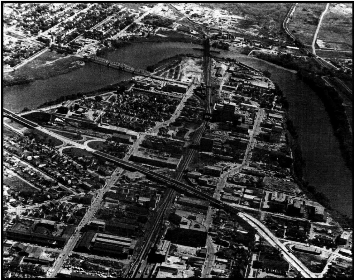
Figure 10. Point Douglas Aerial View, 1960 (Archives of Manitoba, Winnipeg-Views 126).
