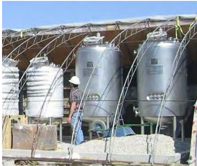
Figure 1.3: Installation of complete mix digesters at Glenlea Research Facility (NCLE, 2008)
