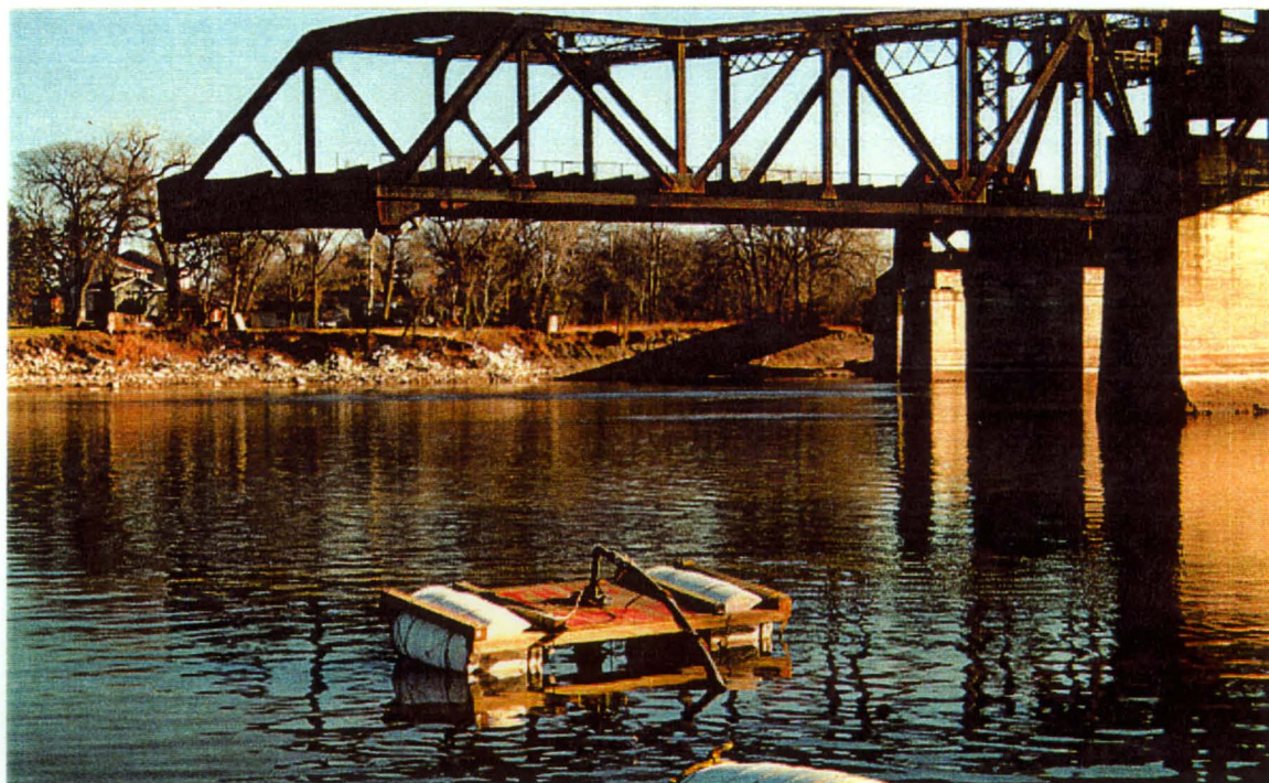
Figure 4-8. Red River water-supply pump.
