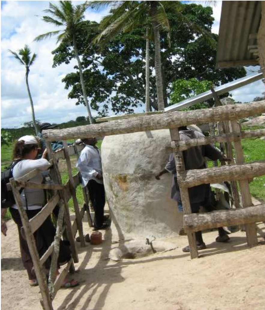
Figure 5.2. Rainwater harvesting using a water jar in Bamba FFS. Water is collected from roof.
