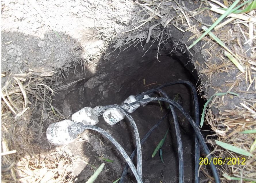
Figure 2.3 Hydra probe installation in the field
