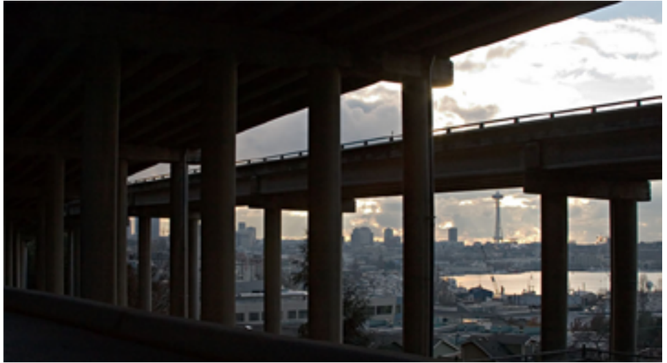
View from under I-5 freeway, 2007.
