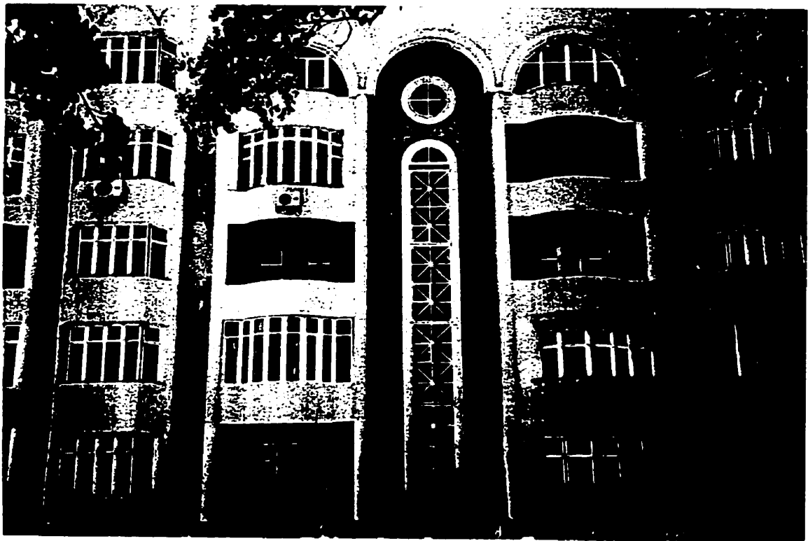
Figure 70. New Apartment Complex - front facade
