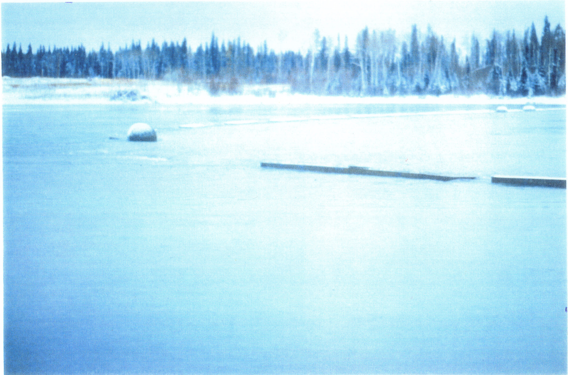
Figure 2 : Section of Jenpeg Ice Boom Submerging Under High Velocity Conditions
