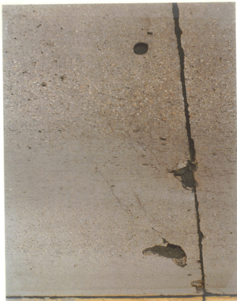
Figure 18: D-cracking on highway 101
