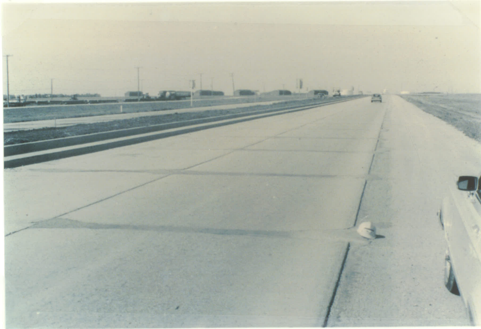
Figure 10: Severe D-cracking on highway 100W 3RB
