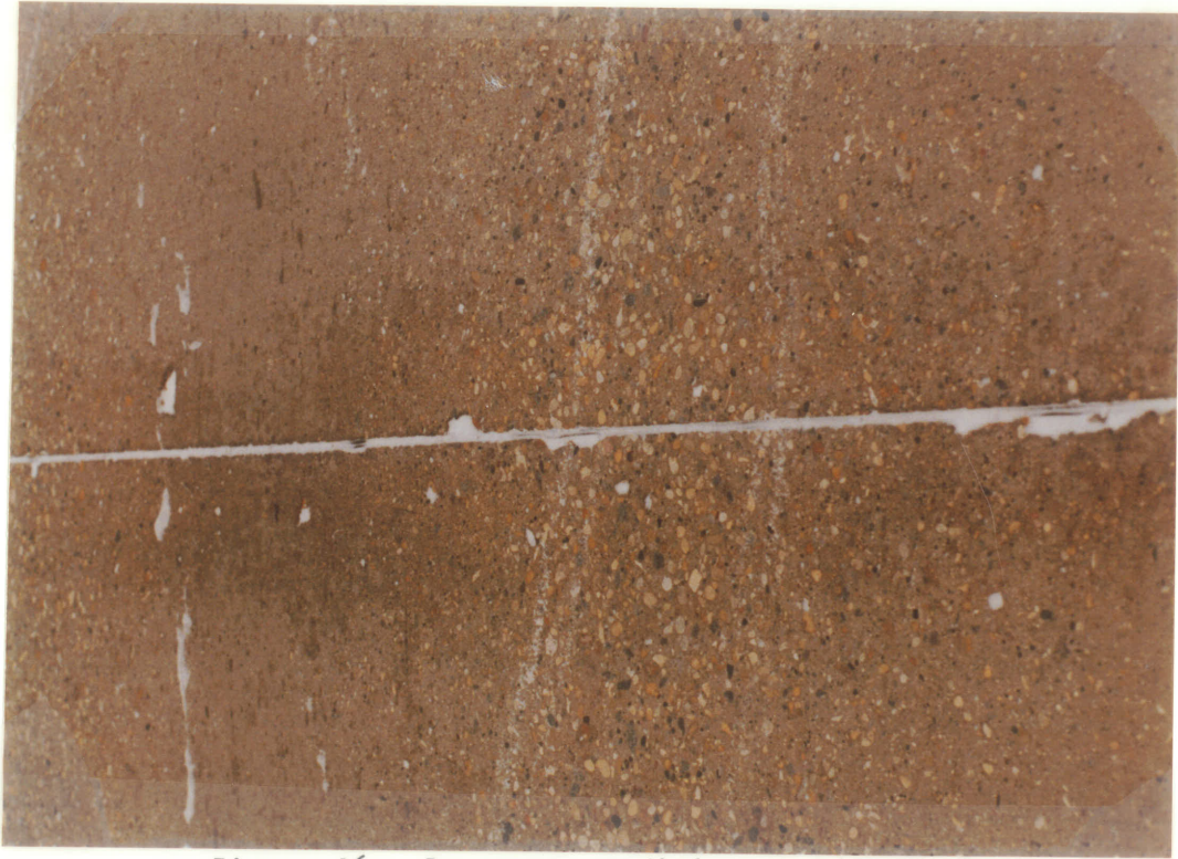
Figure 16: Pavement condition on highway 3
