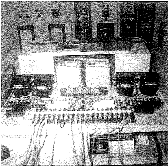
Fig. 14 Power Supplies and Transducers at Kirkfield
