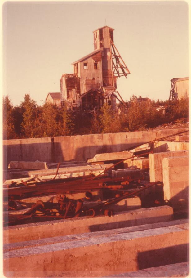
Plate 19: Partial view of the remains of the Gods Lake Gold Mine which ceased its operation in 1945, after a short and unprofitable existence.
