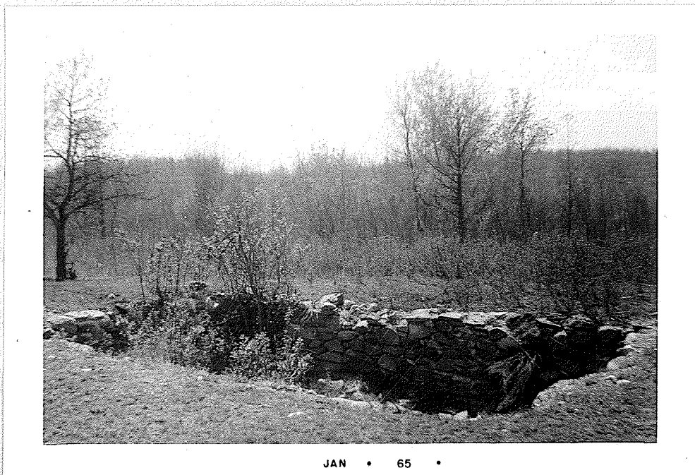
Figure 17 Stones from modified till plain surface deposits used for a house foundation. circa 1700 Location: Along Burrough's Trail Section 1, Township 18, Range 14.
