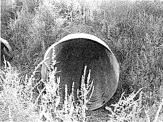
Photos 2: Damage Level 1 – Culverts possessing a large portion of rust.
