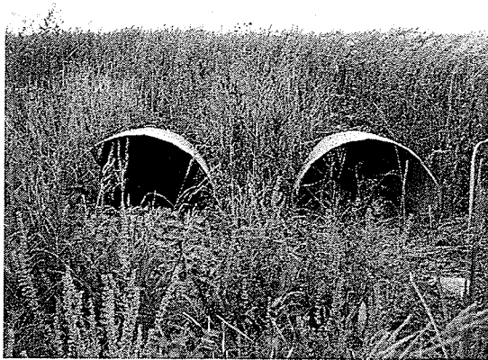
Photos 4: Damage Level 3 – Culverts that are compressed throughout their length.
