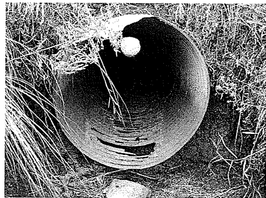
Photos 5: Damage Level 4 – Culverts that had large dents, tears and or holes.
