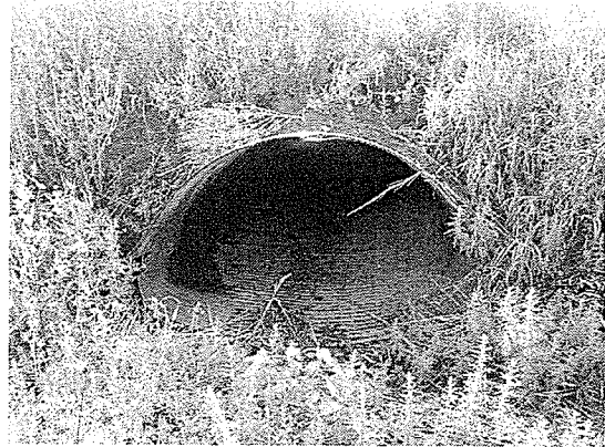
Photos 4: Damage Level 3 – Culverts that are compressed throughout their length.
