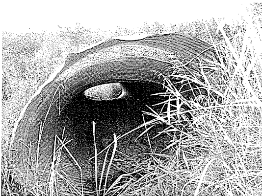
Photos 5: Damage Level 4 – Culverts that had large dents, tears and or holes.
