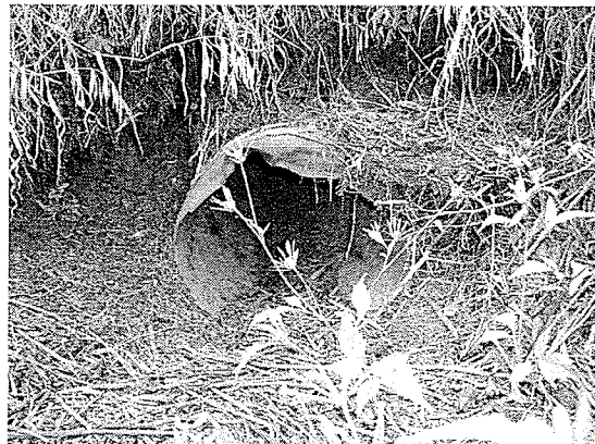
Photos 3: Damage Level 2 – Culverts possessing small dents, tears, and or holes.
