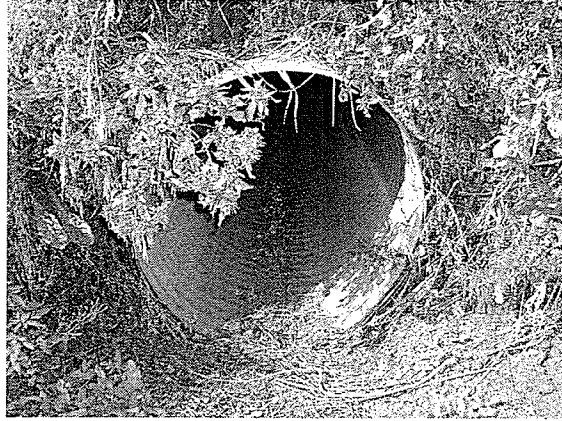
Photos 1: Damage Level 0 – Culverts possessing minimal visible damage.
