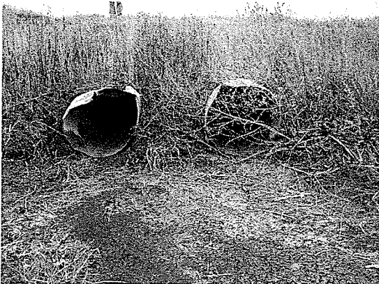
Photos 3: Damage Level 2 – Culverts possessing small dents, tears, and or holes.
