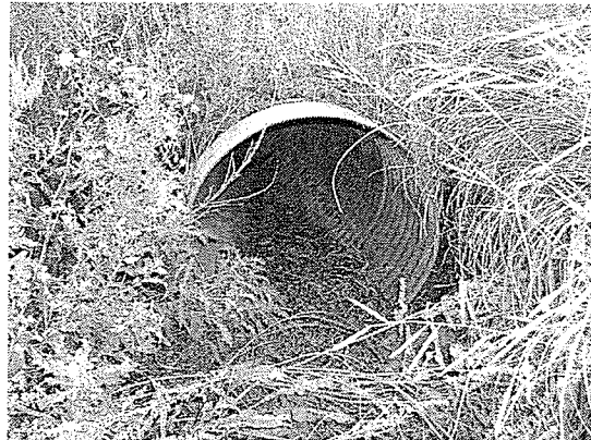
Photos 2: Damage Level 1 – Culverts possessing a large portion of rust.
