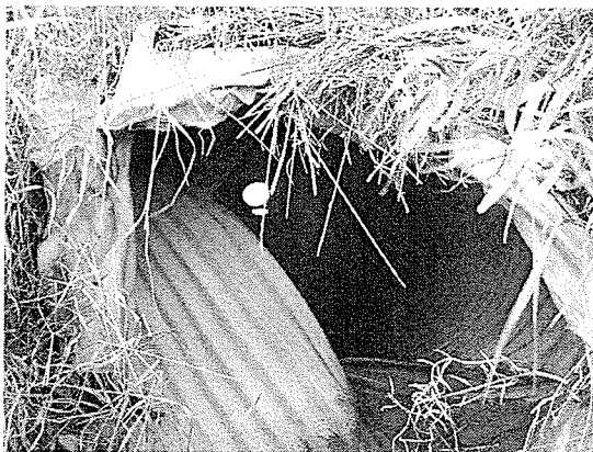
Photos 6: Damage Level 5 – Culverts that were mangled and could impede flows.
