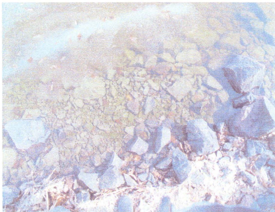
Fig 1.1b “Old” rip rap (site 6). Granite stone installed c . 1970-1980s. Note smaller size of rock (compare to toe of rubber boot at extreme bottom edge of photo) and presence of large gravel “scree” at water’s edge forming the toe of the armouring.
