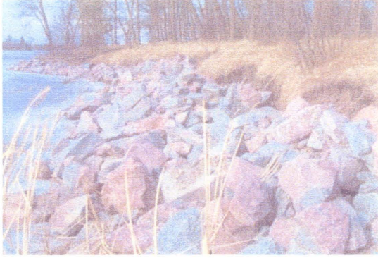
Fig 1.1a. “New” rip rap (site 10). Granite stone installed on shoreline c 2000-2001. Average size of rock approx. 30-60 cm
