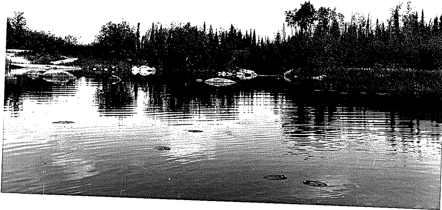
The uppermost dam on the Echimamish. Its initial construction dates back to the early 19th century.
