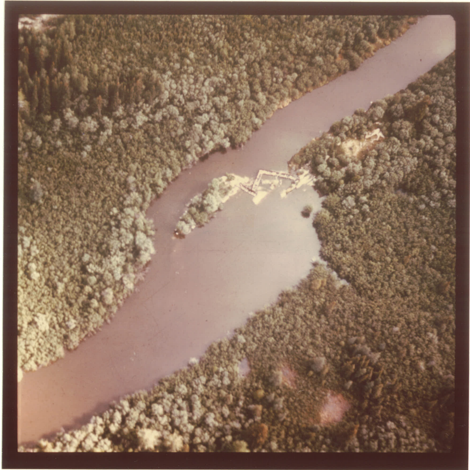
Dam No. 4 was built in the fall of 1936 to assist in the transportation of mining exploration machinery. It is located about 6 miles upstream of Hairy Lake. (Photo courtesy of R. W. Newbury)
