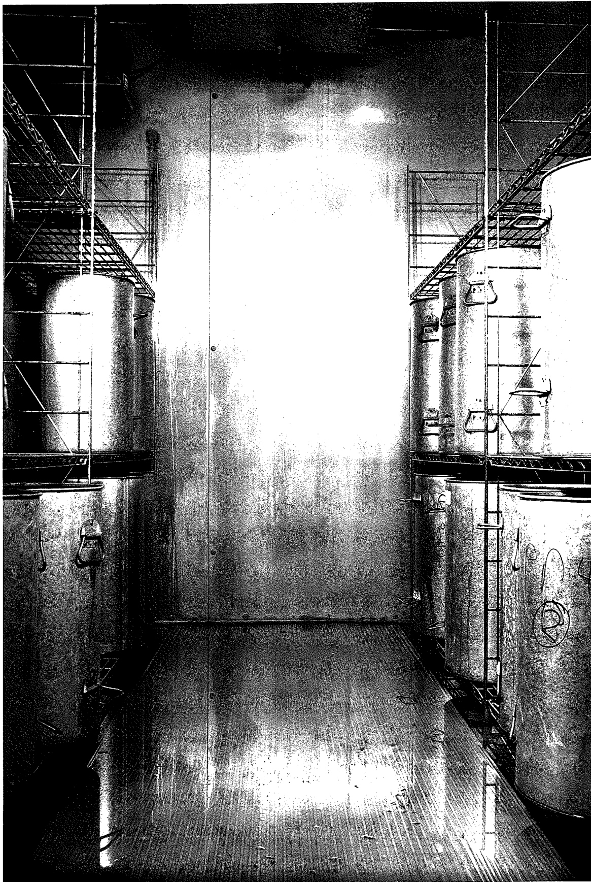
Figure 4. An Interior View of the Cabin
